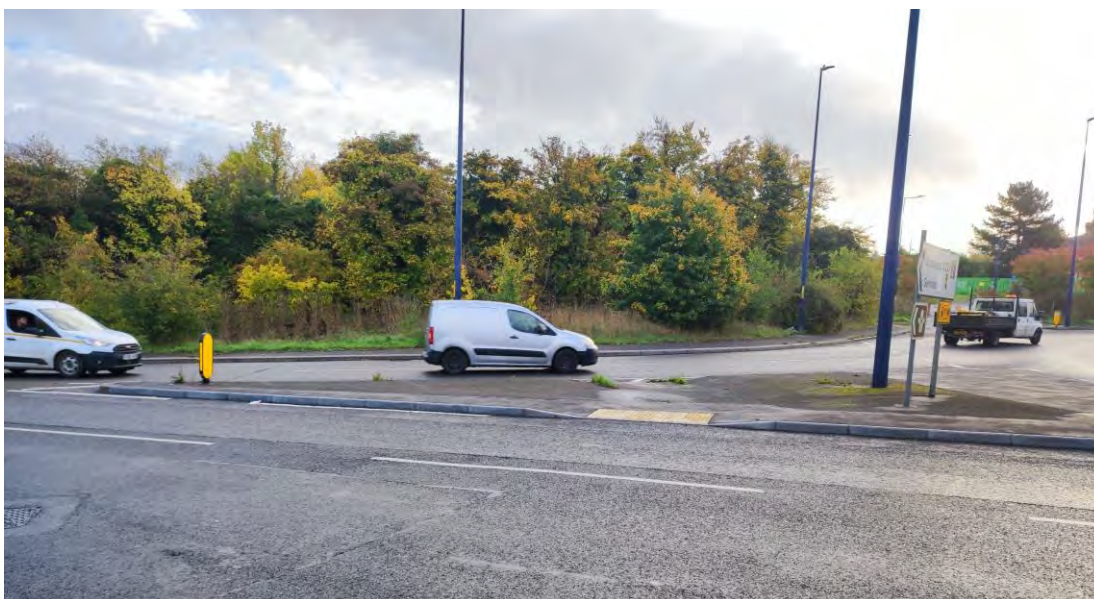
Figure 3.7 A227 (North) – Pedestrian Refuge Island
