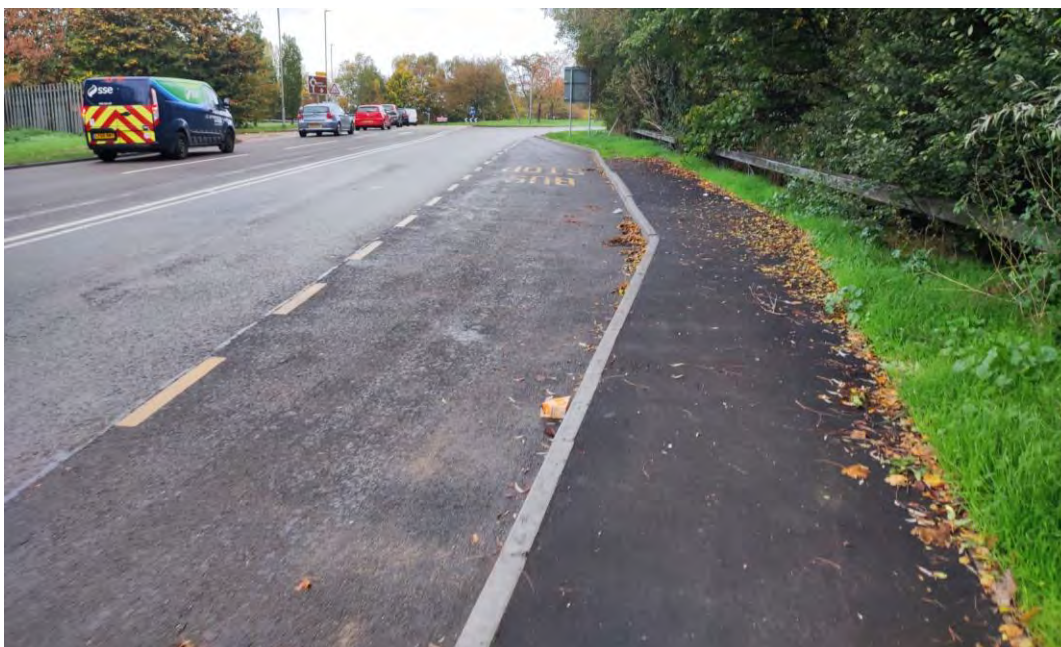
Figure 3.8 A227 (North) – Southbound Bus Stop Improvement
