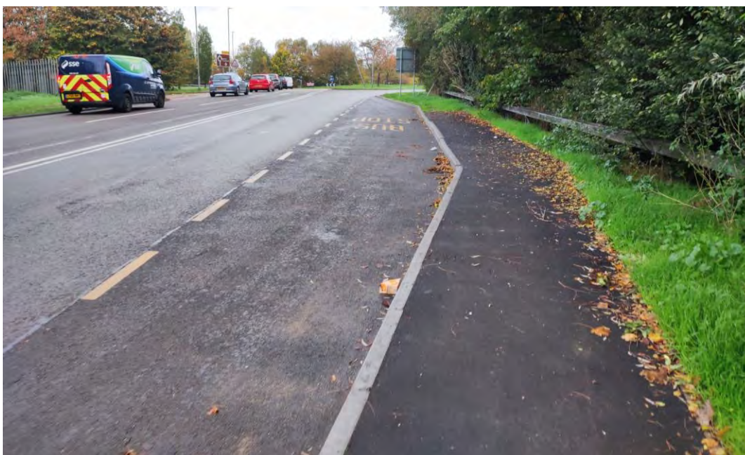
Figure 3.7 A227 (North) – Southbound Bus Stop Improvement
