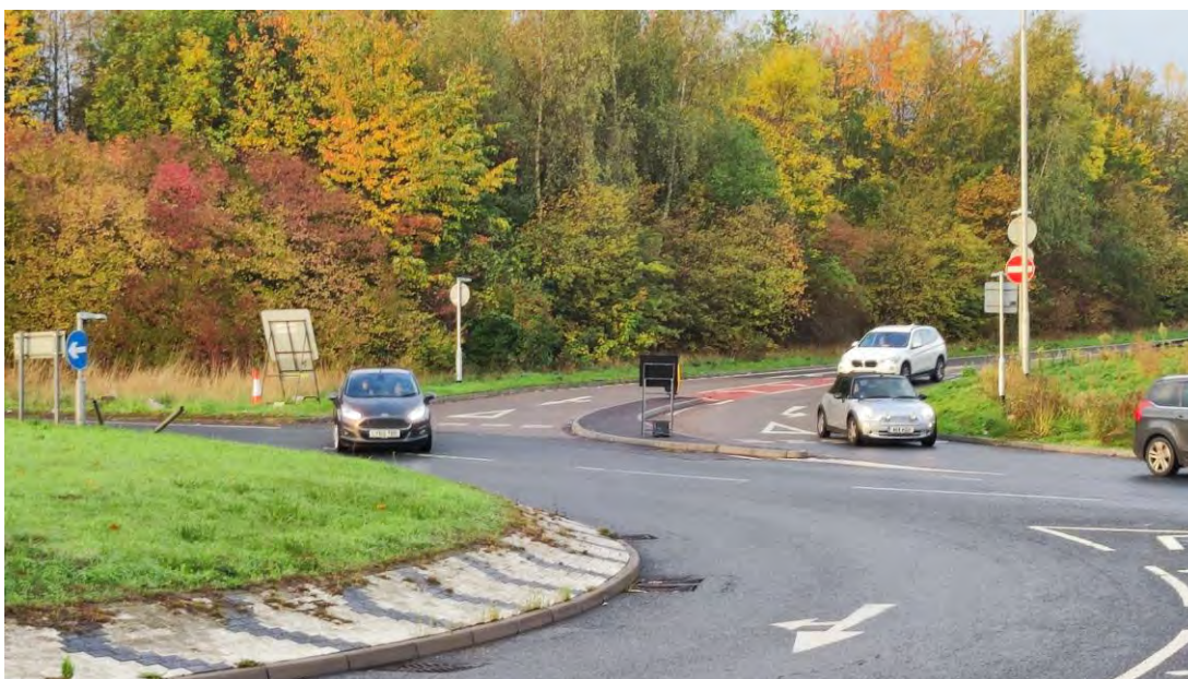
Figure 3.6 A2 Eastbound Off Slip – Highway Improvement
