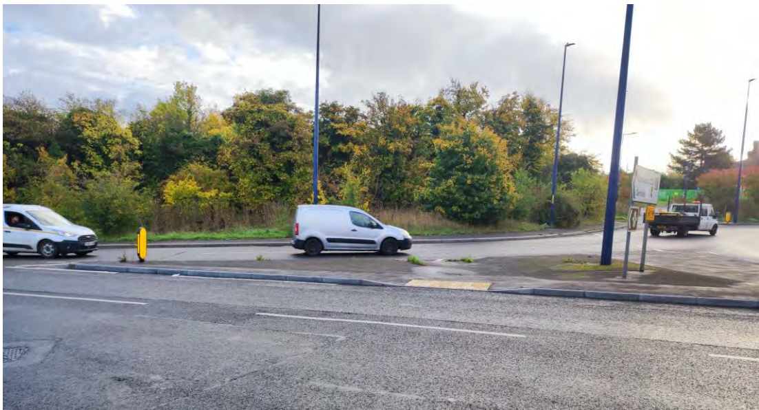
Figure 3.6 A227 (North) – Pedestrian Refuge Island
