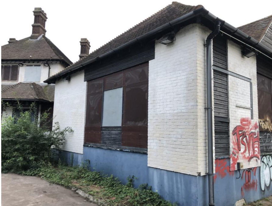
VP2 further view of original hotel facility buildings with floodlighting to roof soffit.
