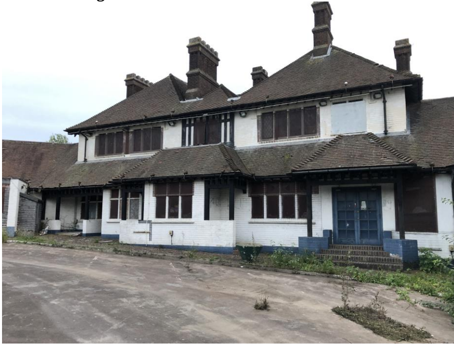
VP1 view to front of hotel original main admin and facility buildings with significant floodlighting at roof soffit level.
