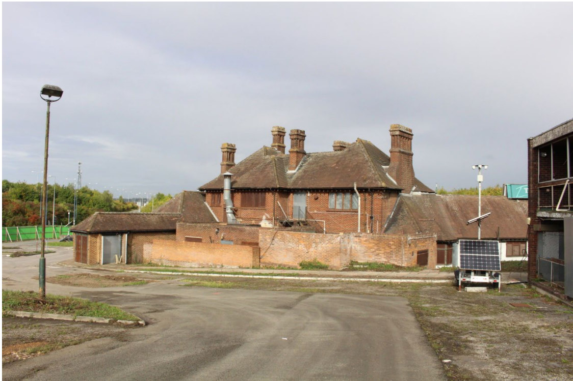
Image EDP 4.4: View of southern side of the building looking north-west, showing the 1970s flat roofed extensions.
