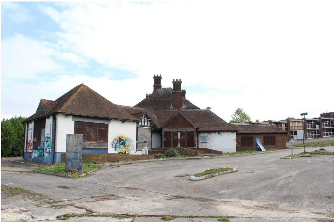
Image EDP 4.6: View looking north-east showing the western wing and 1990s entrance section.
