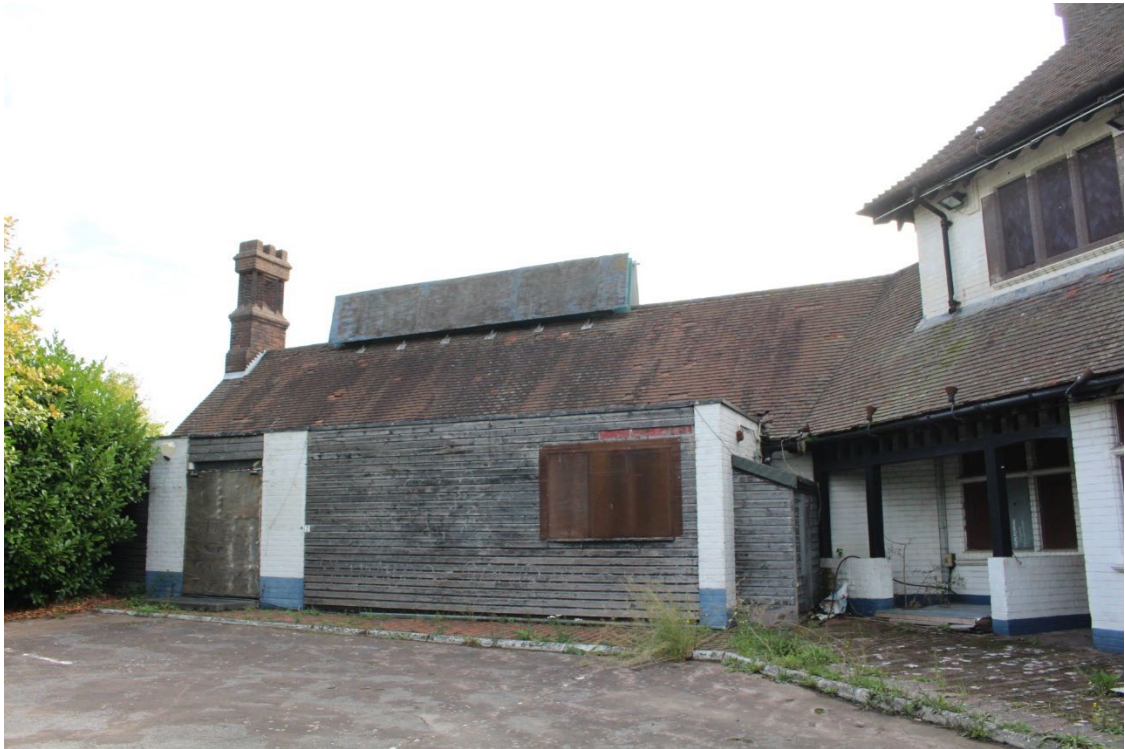
Image EDP 4.5: View of the northern wing looking east, showing the flat roofed extension on its western elevation.
