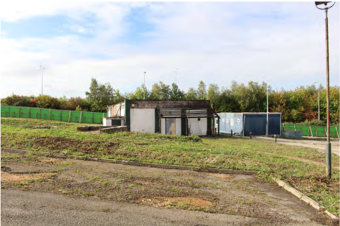
Image EDP A1.3: View of the two buildings in the centre of the site looking south, showing the building platforms terraced into the slope.
