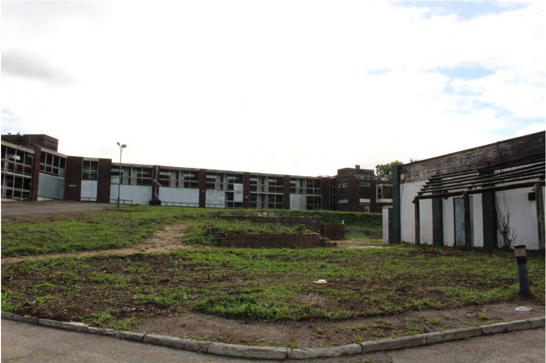
Image EDP A1.4: View of the centre of the site looking east, showing the terracing in this part of the site and the 1970s motel building built on a level platform.
