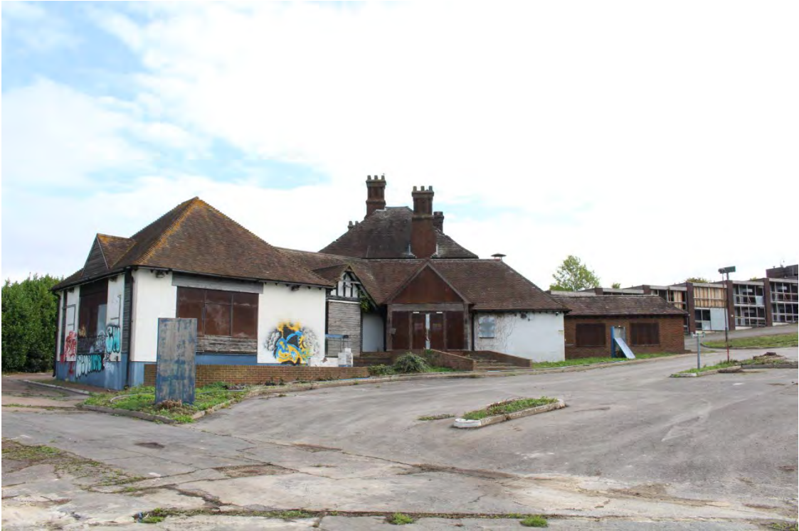
Image EDP A1.2: View of the much-altered 1920s building showing how it is terraced into the slope, looking north-east.
