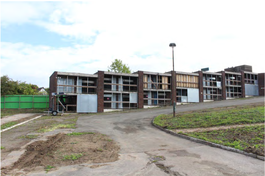
Image EDP A1.5: View north of the northern 1970s block, showing how it steps up and is terraced into the slope.
