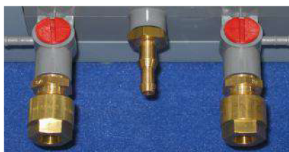
Connections for tubing in different type's available e.g. 8 mm ferrule union
