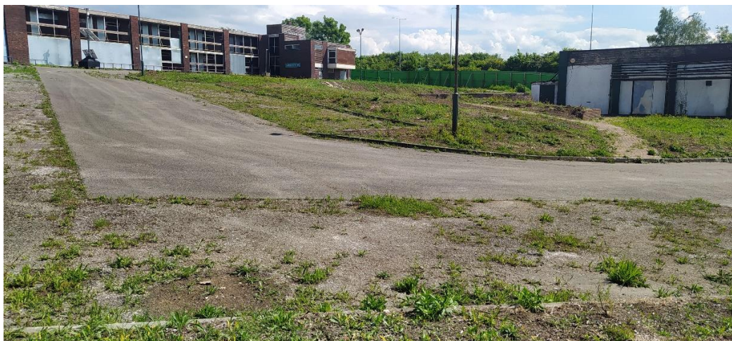
Photo 10 From the centre north looking south-east, showing buildings (B2 and B3), developed land sealed surface and ruderal / ephemeral (centrally) (2022)
