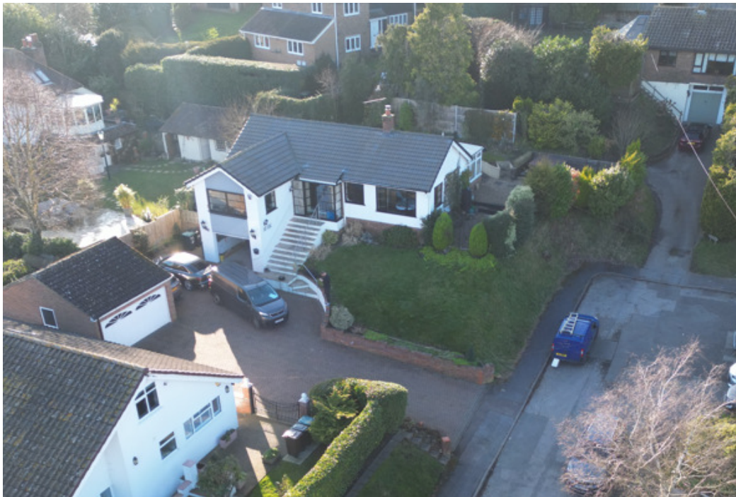
P003 – aerial view of site looking west
