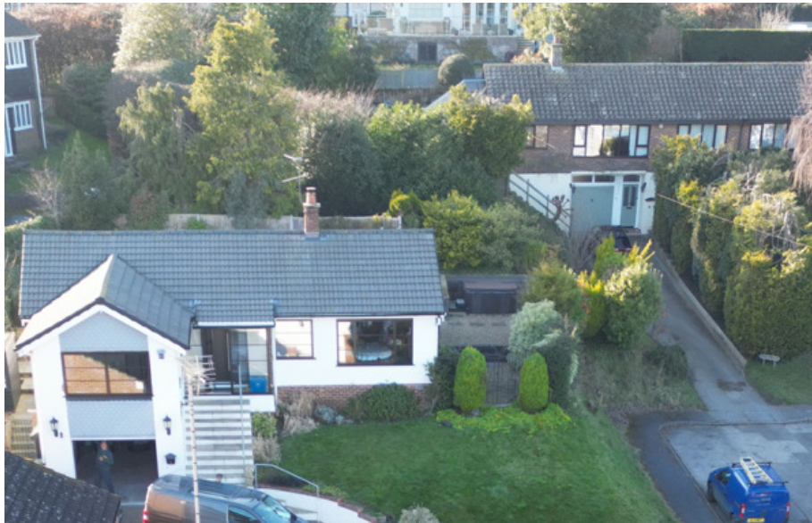
P005 – site context looking westerly
