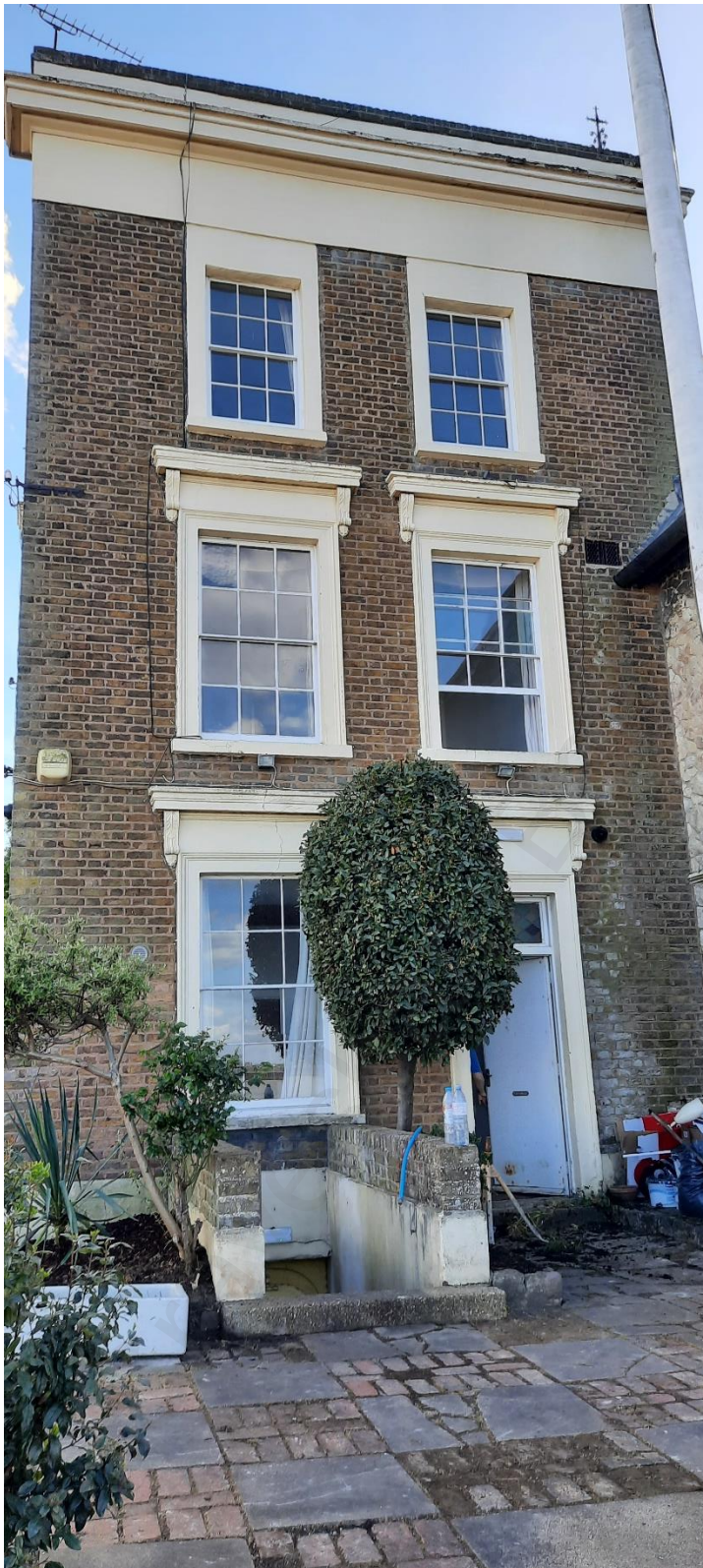
Photograph 1: Rear Elevation (north facing elevation). No Change resulting from the proposal
