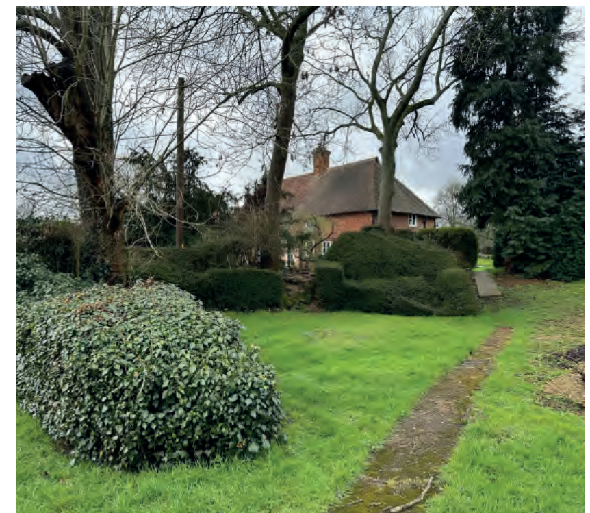
5. View of Boughurst Farm House north east at end of driveway.
