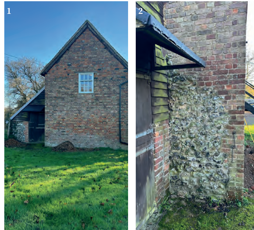
1. Rear lean-to in flint with modern roofing sheet. 2. Brickwork and flint stitched together.
