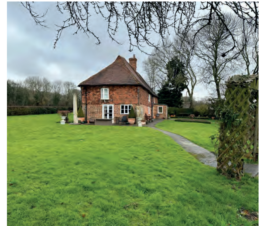
2. View of Boughurst Farm House from the south.
