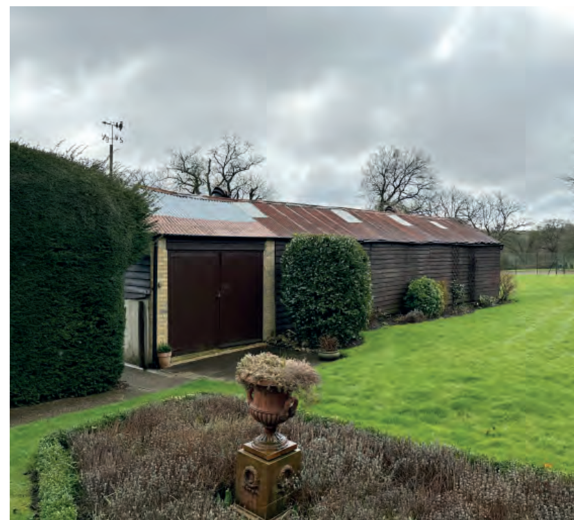
4. View of outbuildings, west side.
