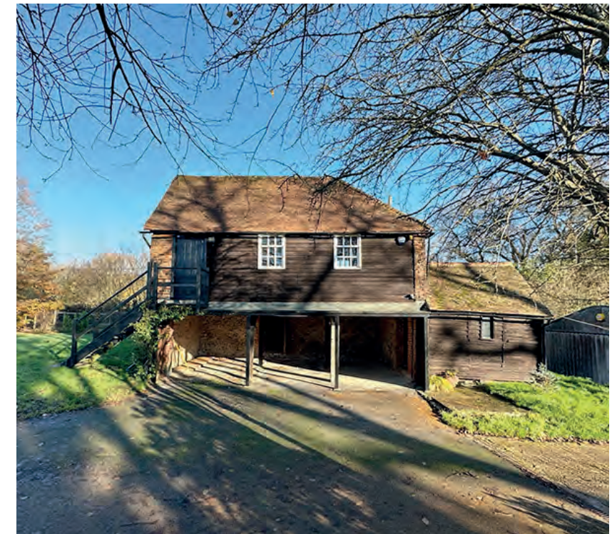
2. West elevation (front) of the gatehouse.
