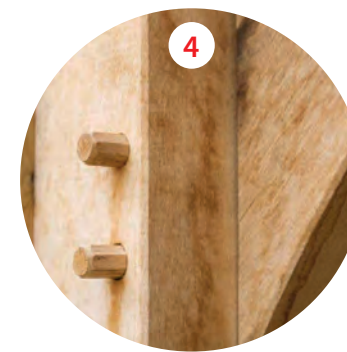
Oak framing with traditional details (to car parking bays)
