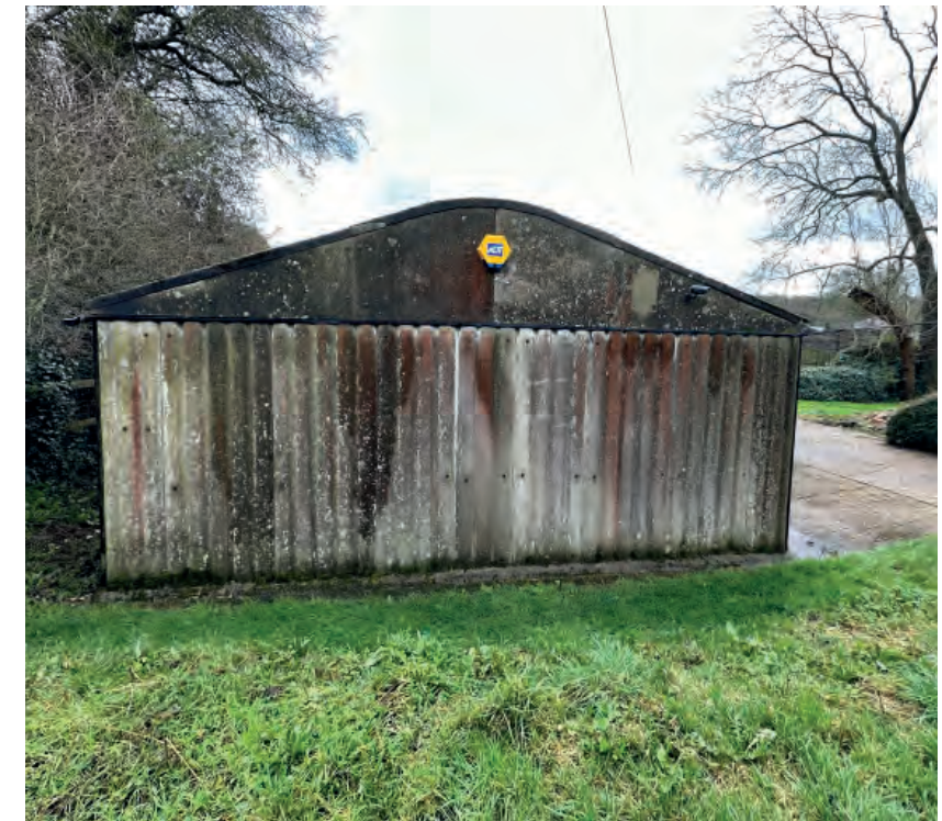
2. Modern workshop/store west elevation.
