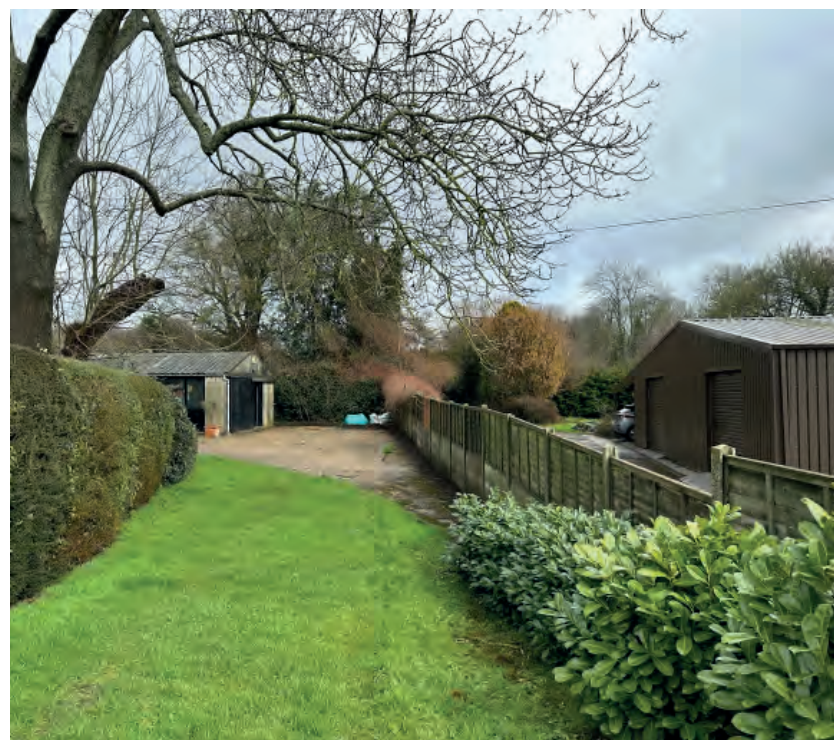
3. Workshop/store distant approach from the south.
