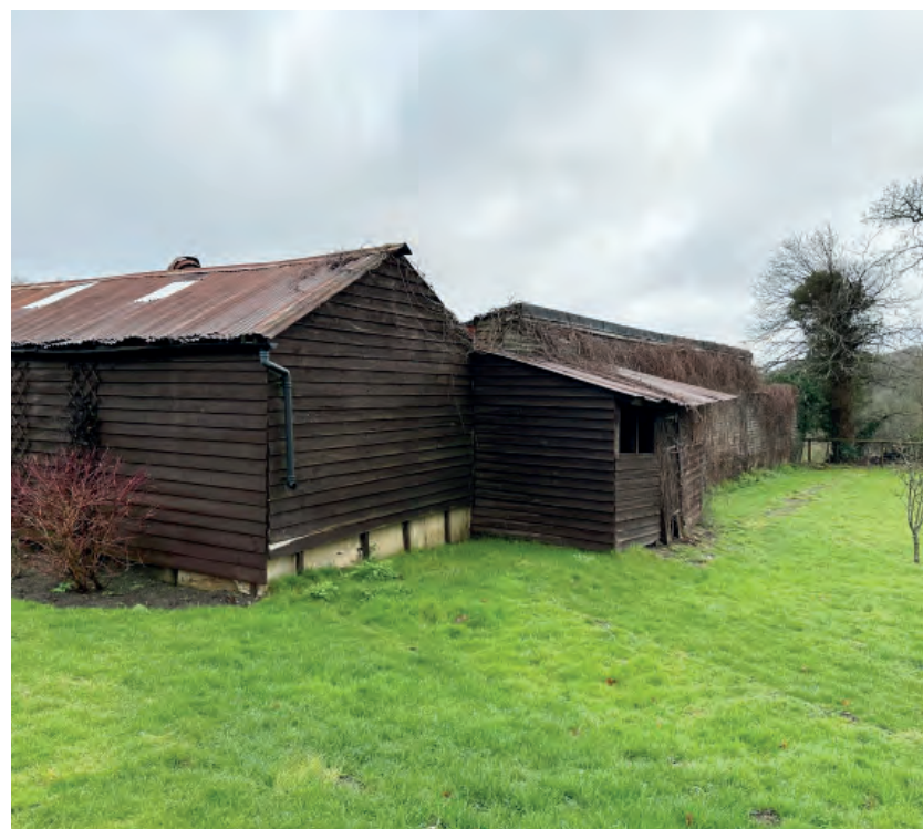
3. View of outbuildings (partially derelict), south side.
