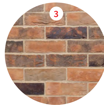
Brickwork (to plinth)
