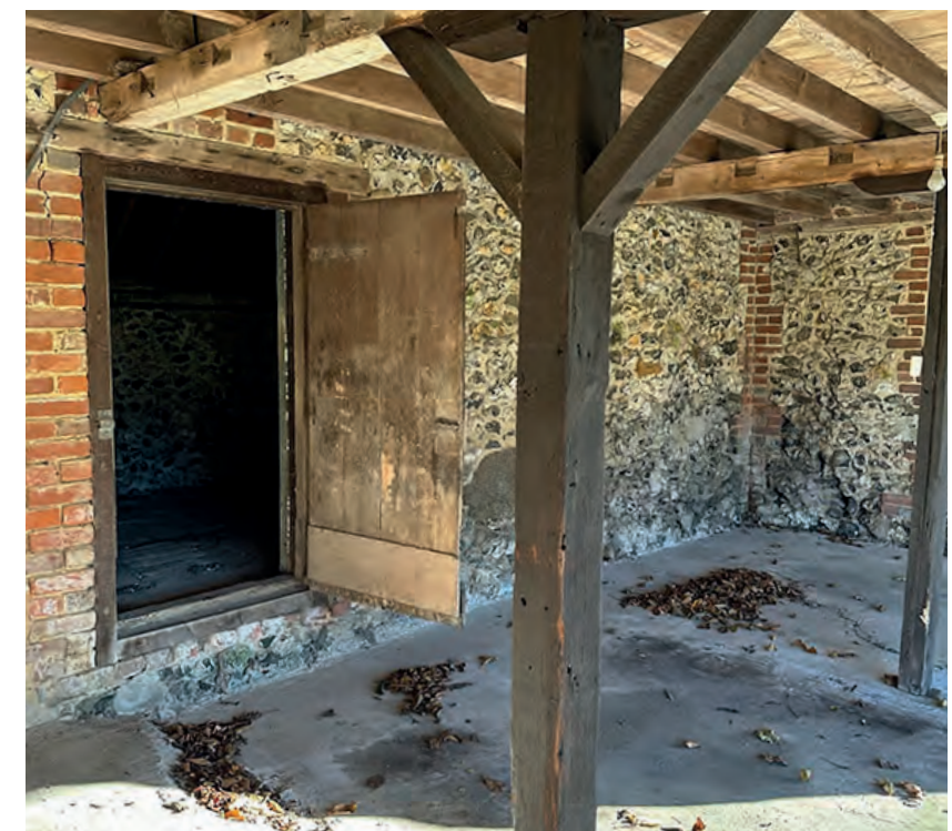
4. Current parking area, mix of flint and brickwork to walls.
