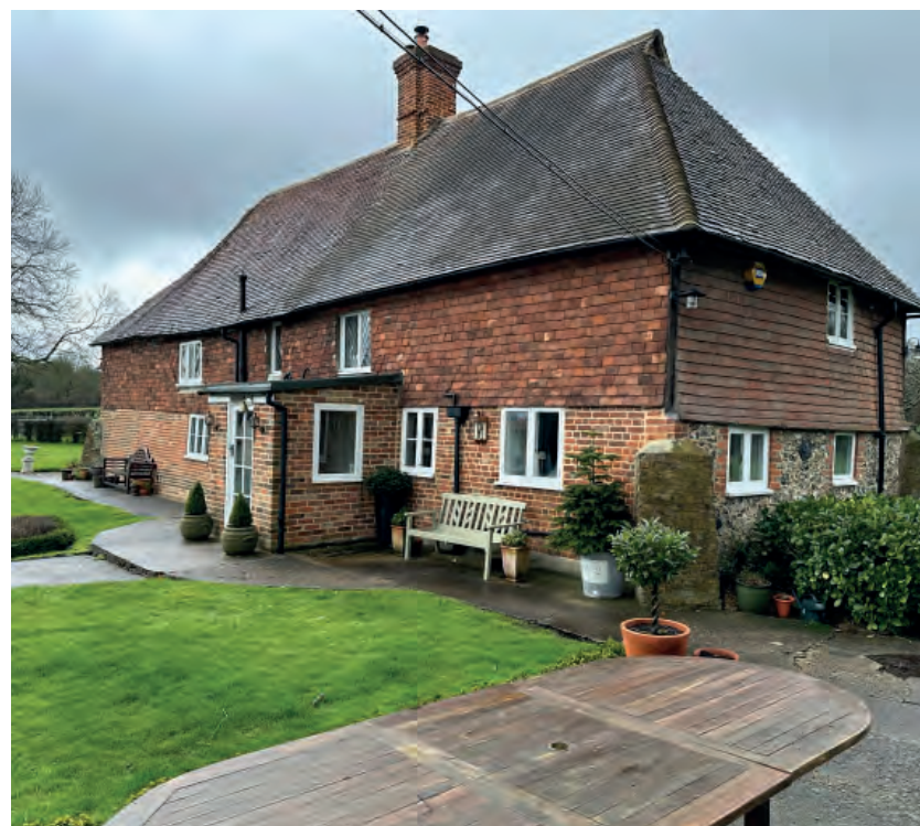
3. View of Boughurst Farm House from the north east.
