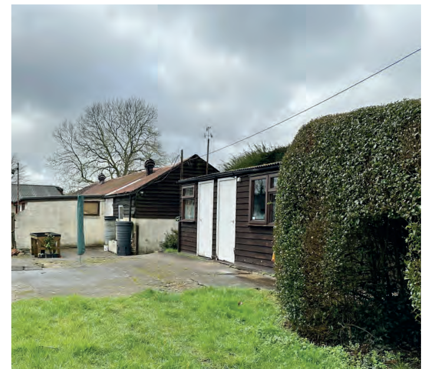
5. View of utility building.
