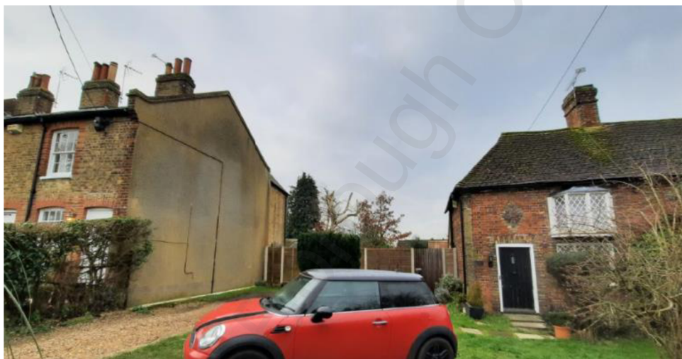
Figure 2: Front Elevation of 3 Park Cottages (on right of image); 12 Homewood Cottages (on left of image)
