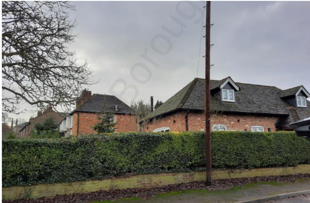
Figure 5: View of Chestnut Green Cottage (foreground) and Side Elevation of 1 Park Cottage (background) with Homewood Cottages beyond. Photograph taken from Racefield Close.
