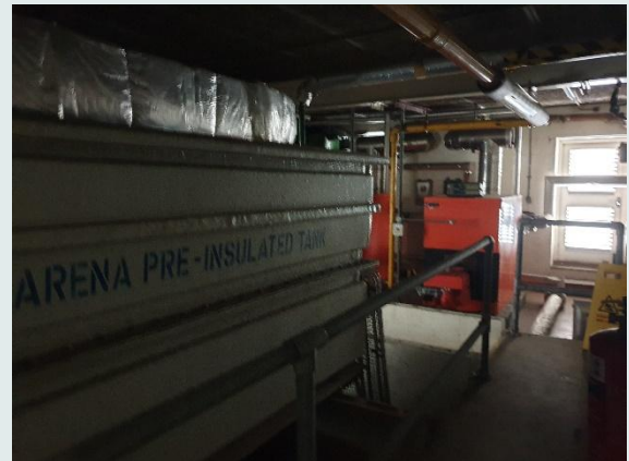
Plant room on roof
