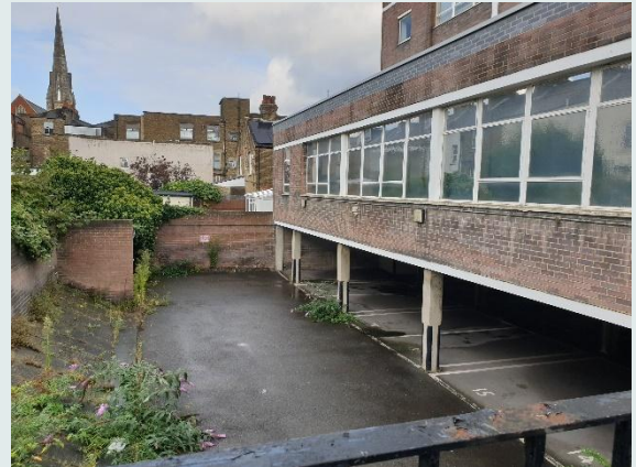
Open-sided undercroft car park and rear extension
