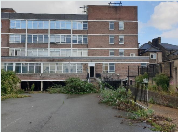
Rear façade of building
