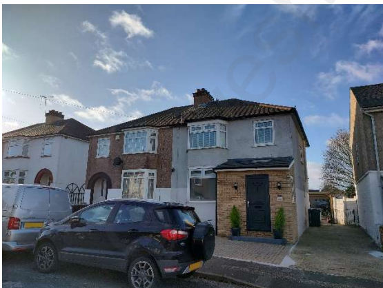
Fig 3. Photo to the front
