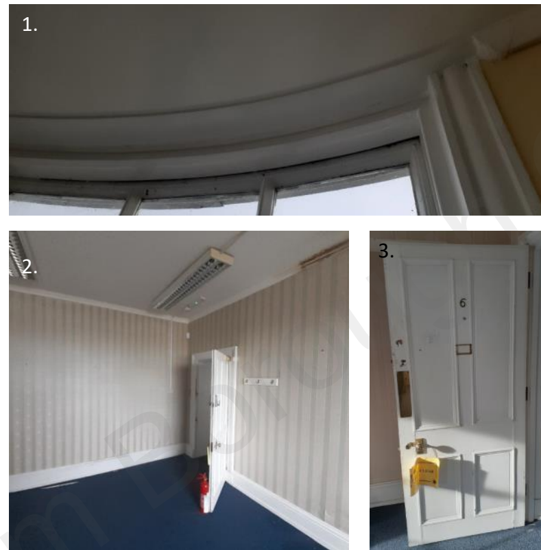
1. Coving detail: 2. ceiling with coving: 3. original internal door
