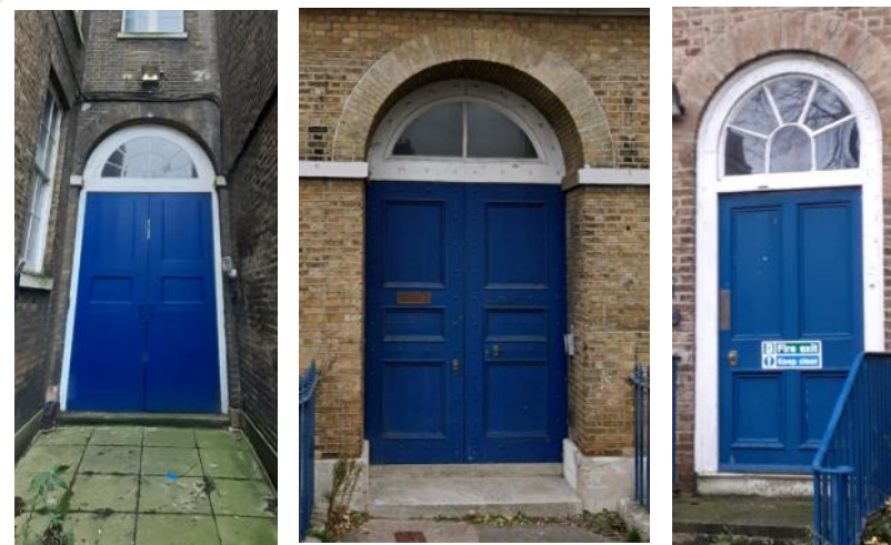
External doors to be refurbished and retained.
