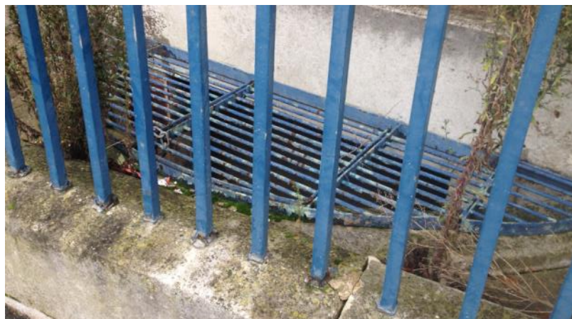
Photo of front elevation light well
