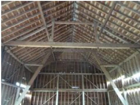
3. Image above shows the underside of the roof structure.
