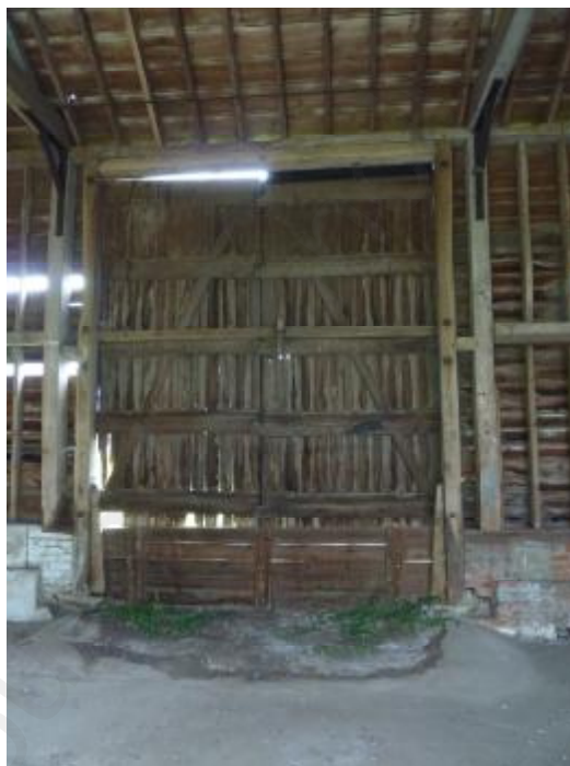
Fig.5 – Parsonage Barn doors
