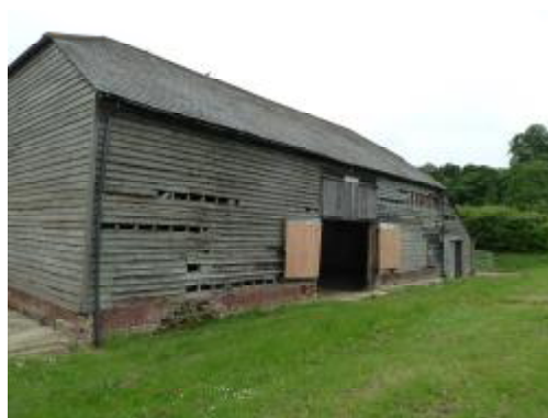
12. View from the West with half of the barn doors open.
