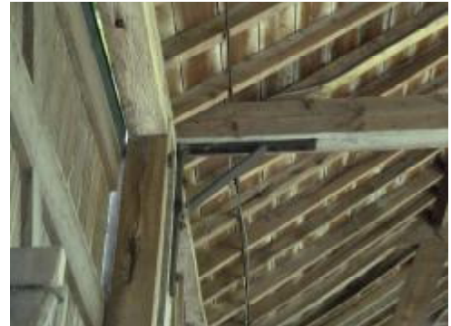
2. Image above shows a recent photograph of internal structural frame and truss, next to the door. Most of the structural frame timbers are in good condition.
