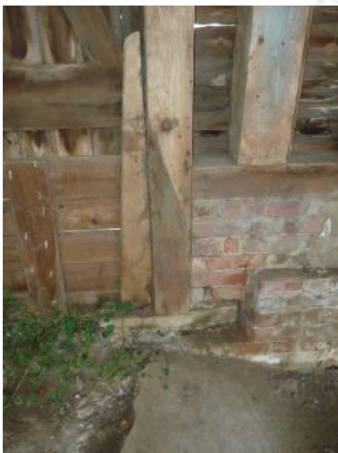
5. Image above shows the brick plinth internally, with door frame post, base rail to timber framing and principal post.
