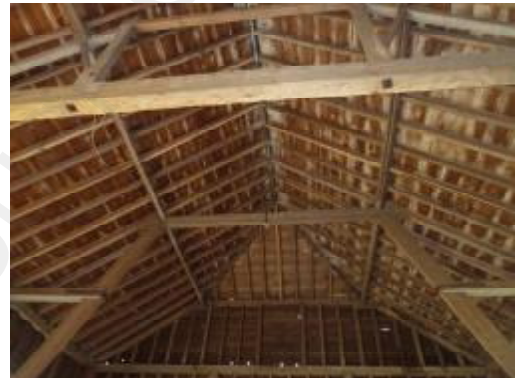
4. Image above shows the underside of the roof structure
