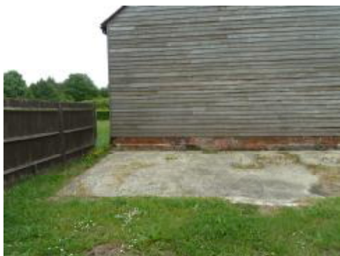
11. South West elevation, showing existing slab which will be removed. This area will house the new extension.
