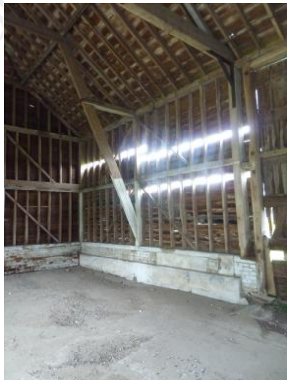
Fig.4 Internal Image of barn structure
