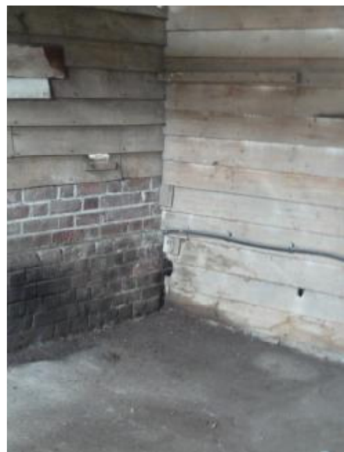
6. Image above shows the brick plinth internally to the garage, with feathered edge cladding above.
