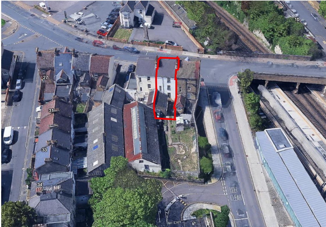
Image 6: Overhead front view of the site (outlined in red) facing east.
