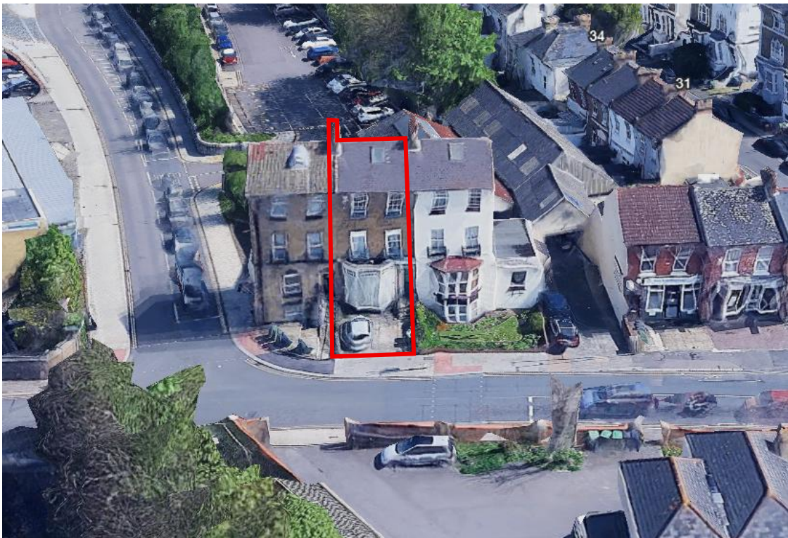
Image 5: Overhead rear view of the site (outlined in red) facing west.
