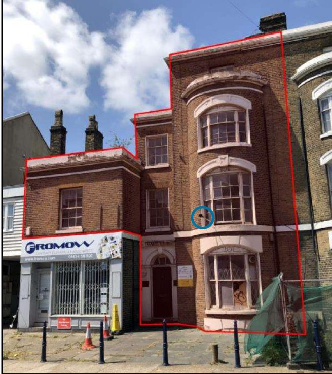
Figure 2.1: Front elevation, extent of properties (red) (Google Maps ®) and external noise monitoring location at 1 st floor level (blue)
