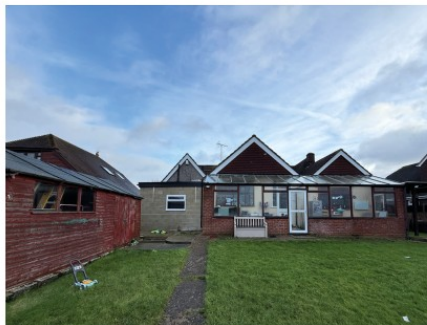
Fig.4 - Rear elevation of site showing existing extension
