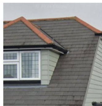
Slate Roof Hips/Dormers on Lewis Rd
