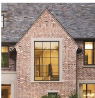
Stone Surround to Aluminium Windows
