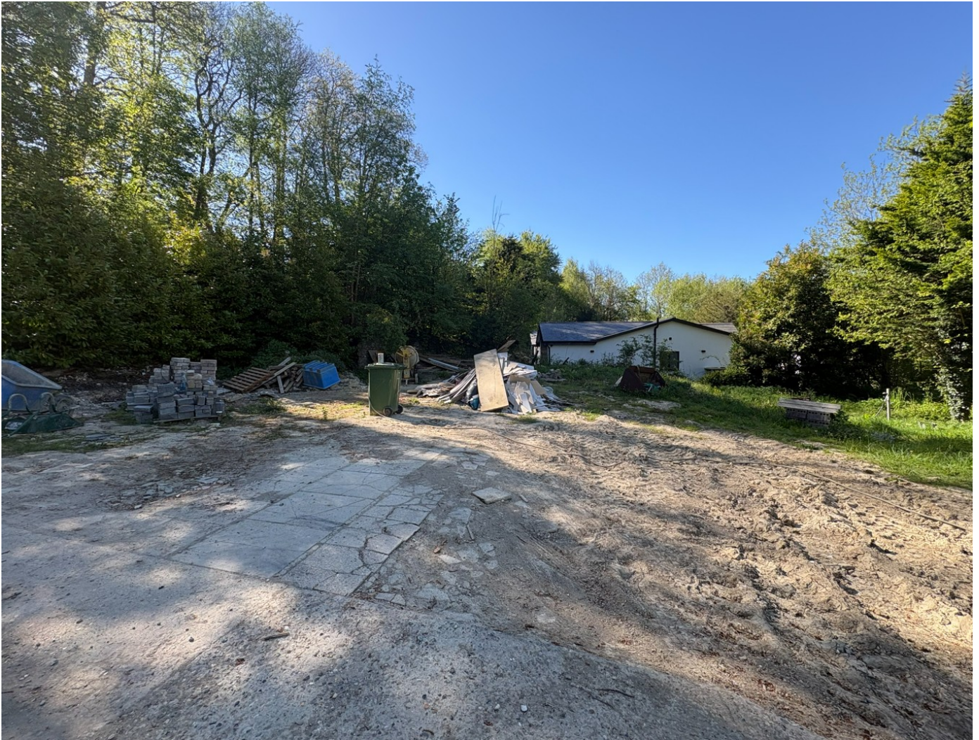
Image taken during site visit of the area where the garage would be built
