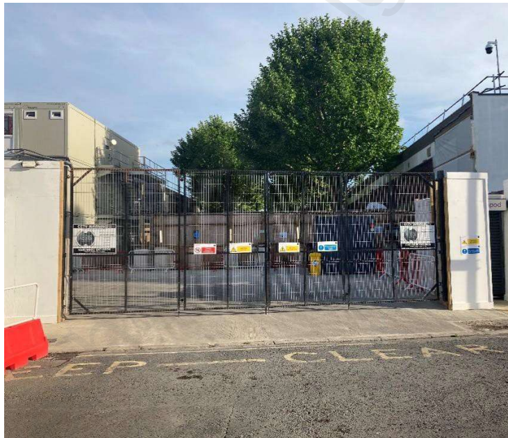
Figure 1 – typical site entrance
