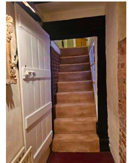
inserted C19th stair and door to be removed viewed from living room
