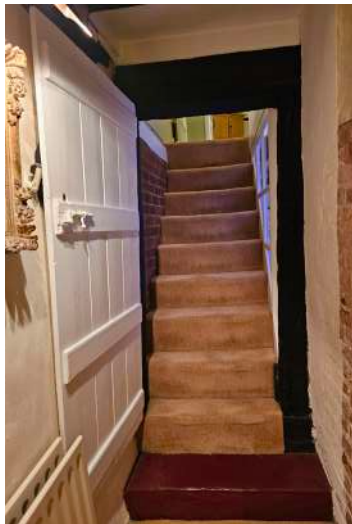
stair and door to be removed
