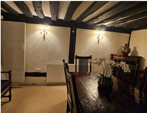
south bay (solar?) showing possible end jetty joist orientation
