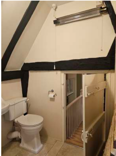
bathroom to west showing link through to north bays under closed truss with no double post or recessed bay indicative of Wealden type frame
