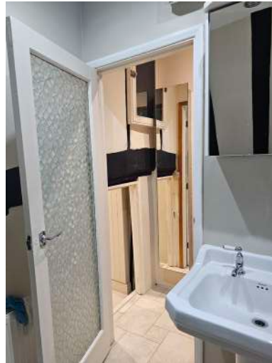
inner corridor showing low doorway under tie beam to open truss with modern partitions to bathroom
