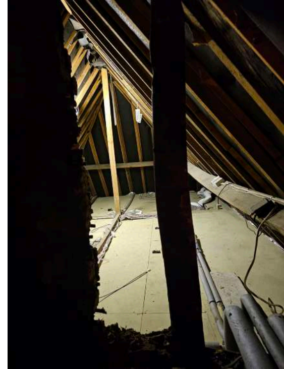
modern softwood roof frame to northern 2 bays with daubed smoke-blackened partition behind chimney indicating former floored partition
