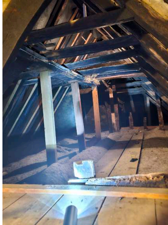
southern bays showing (propped) collar purlin and smoke blackened timbers and daub to solar chamber indicative of former full open hall
