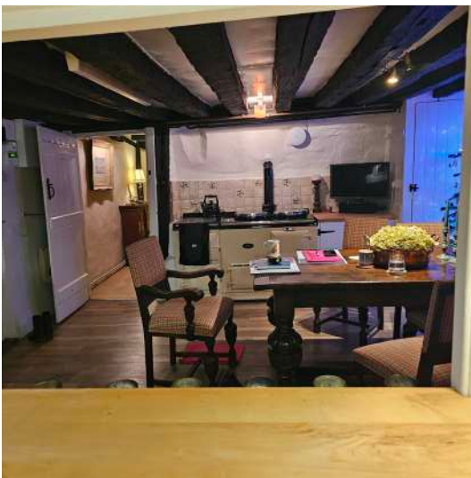
dining room - original north end service bay and altered fireplace
