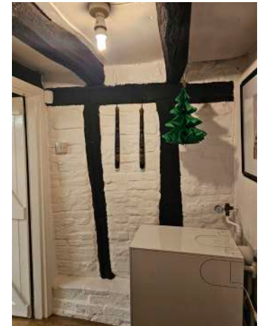
utility room - external face of original north external wall with end jetty possibly lost. Note plinth
