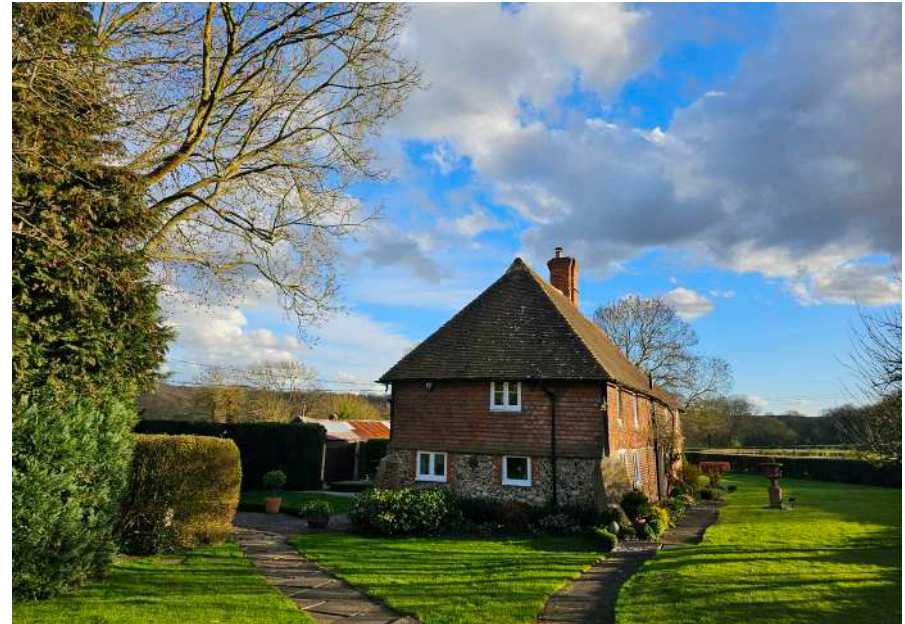
north elevation of house
