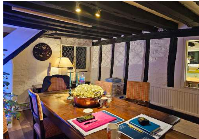
dining room - original north end wall frame. Note mortices in central joist and scar on plaster near window suggestive of earlier door position
