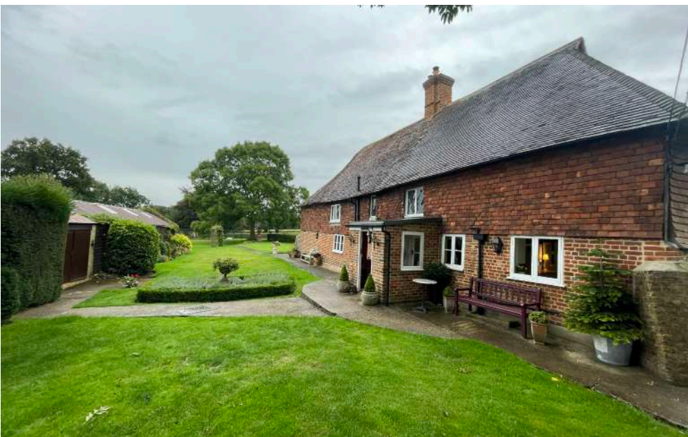
east elevation of house
