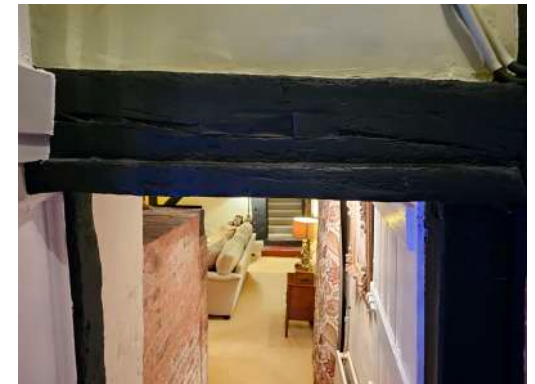
empty mortices for floor joists in inserted circa C19th stair
