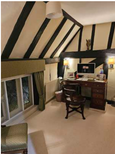
study - showing truss to north/possible smoke bay?
