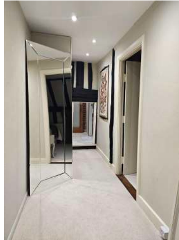
modern partitions of inner corridor showing low doorway under tie beam to open truss
