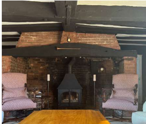
living room - inserted chimney. Note bridging beam supporting spine beam at possible smoke bay/half-floored hall
