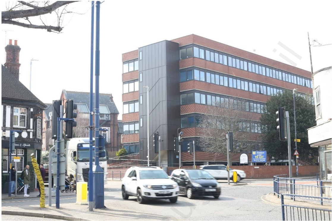
Plate 1 Joynes House, eastern and northern elevations.
