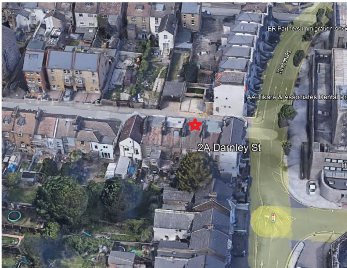
Aerial view of 2A Darnley Street and surrounding area
