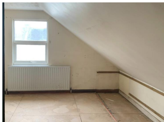
Photograph 04: Existing second floor rear bedroom
