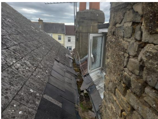
Photograph 03: Existing Roof to 57 Sun Lane
