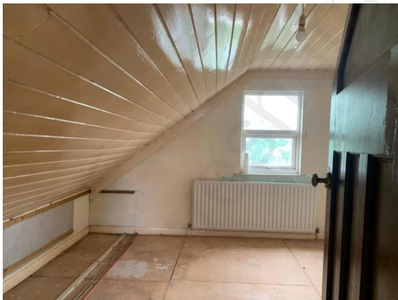
Photograph 01: Existing second floor rear bedroom
