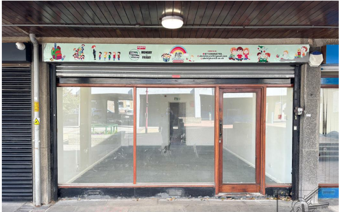
PHOTO ABOVE: FRONT ELEVATION ('SHOP FRONT') AS EXISTING
