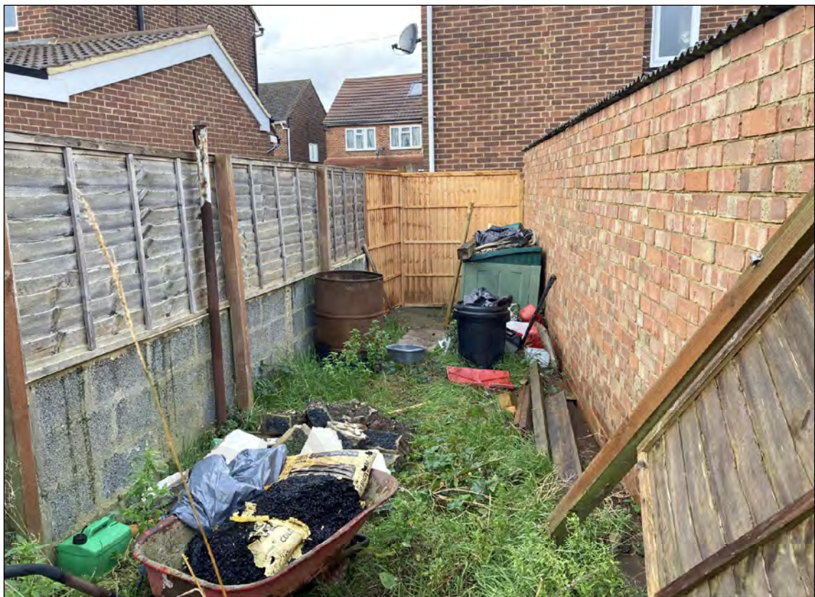
Plate 10: View of the Site extension to the south, looking west
