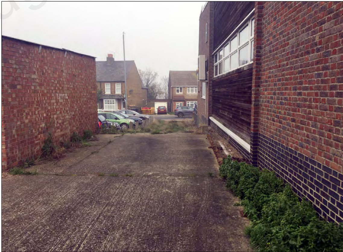
Plate 4: View looking north from within the Site, showing ramp down to Lower Higham Road
