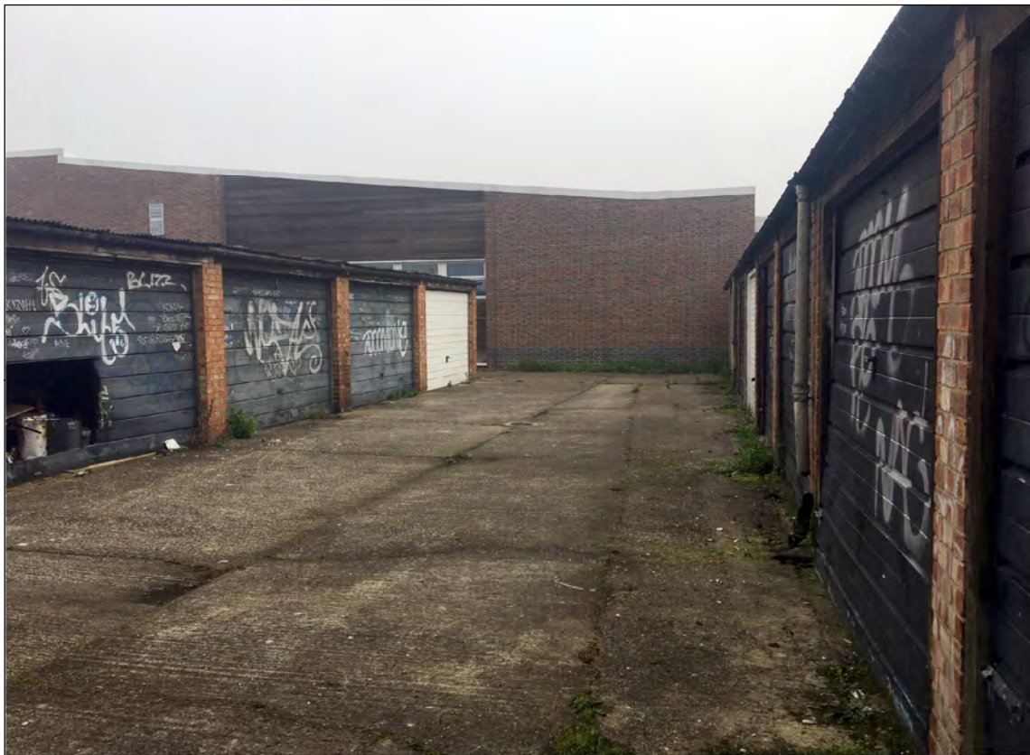
Plate 1: View looking east within the Site from the western Site boundary
