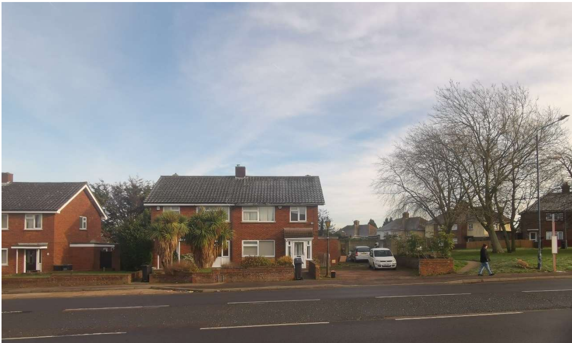
Fig 2.1 Photograph of no 53 Coldharbour Road (note: bus stop to right of image)
