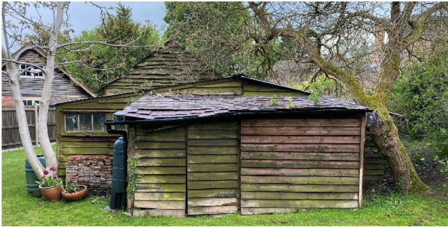
view of the existing north elevation looking south towards the neighbours outbuilding, which is of a similar scale to this proposal. The 2 trees in the foreground are to be removed.
