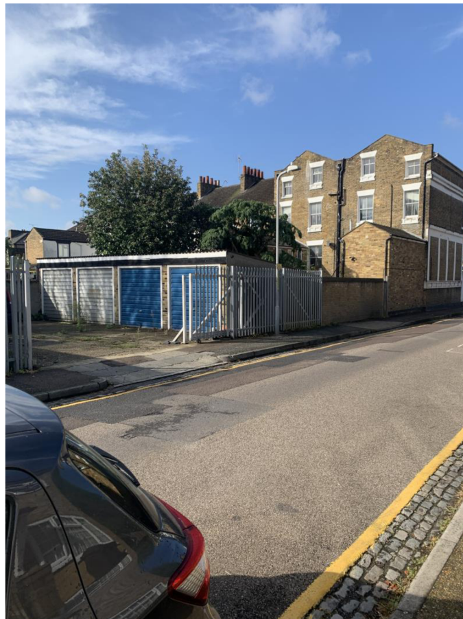
View of existing garages
