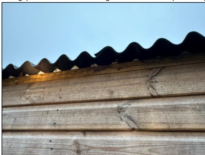
Photo 4.15: The gaps underneath the corrugated roof are filled preventing bat access.
