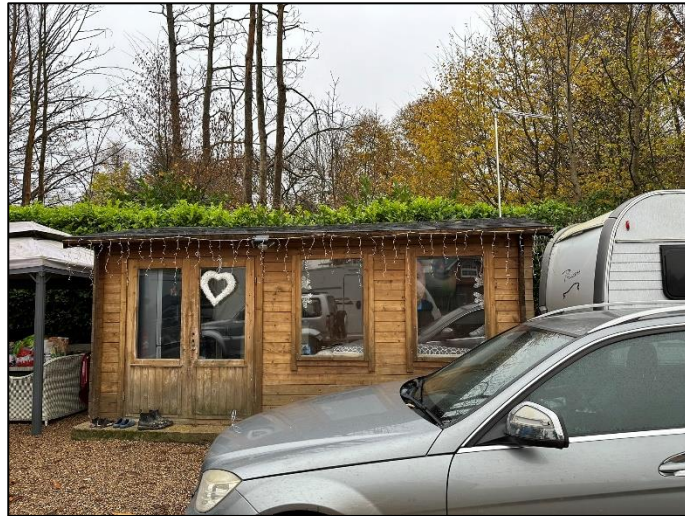
Photo 4.12: The northern elevation of Building B3, facing south
