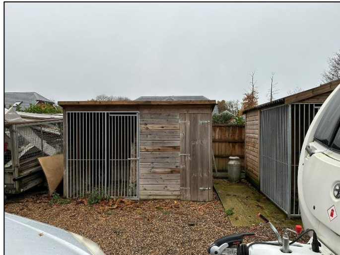
Photo 4.13: The southern elevation of Building B4, facing north.
