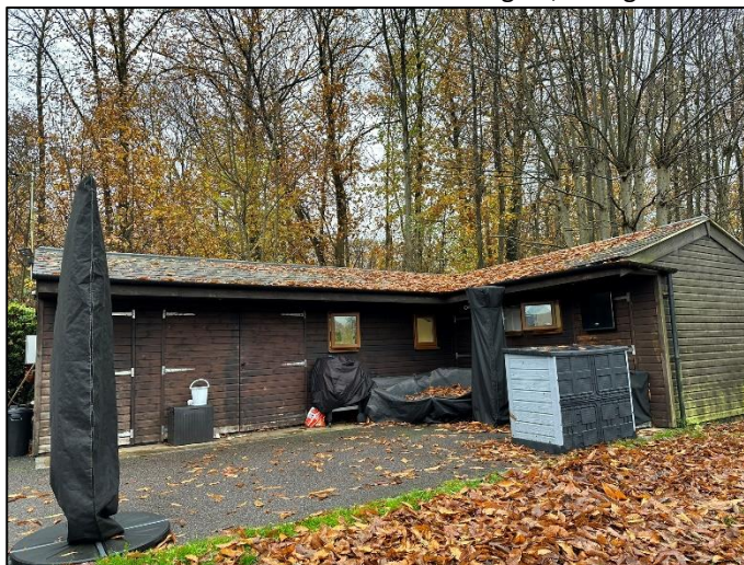
Photo 4.8: The northern elevation of Building B1, facing south-west.
