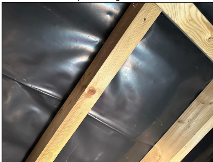
Photo 4.10: The plastic lining and rafters in the loft.
