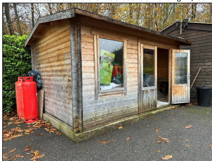
Photo 4.11: The eastern and northern elevations of Building B2, facing south.
