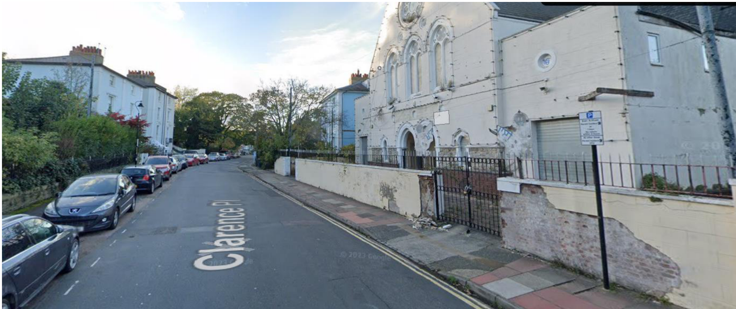
Fig.3. View of the front of the property on Clarence Place looking west.
