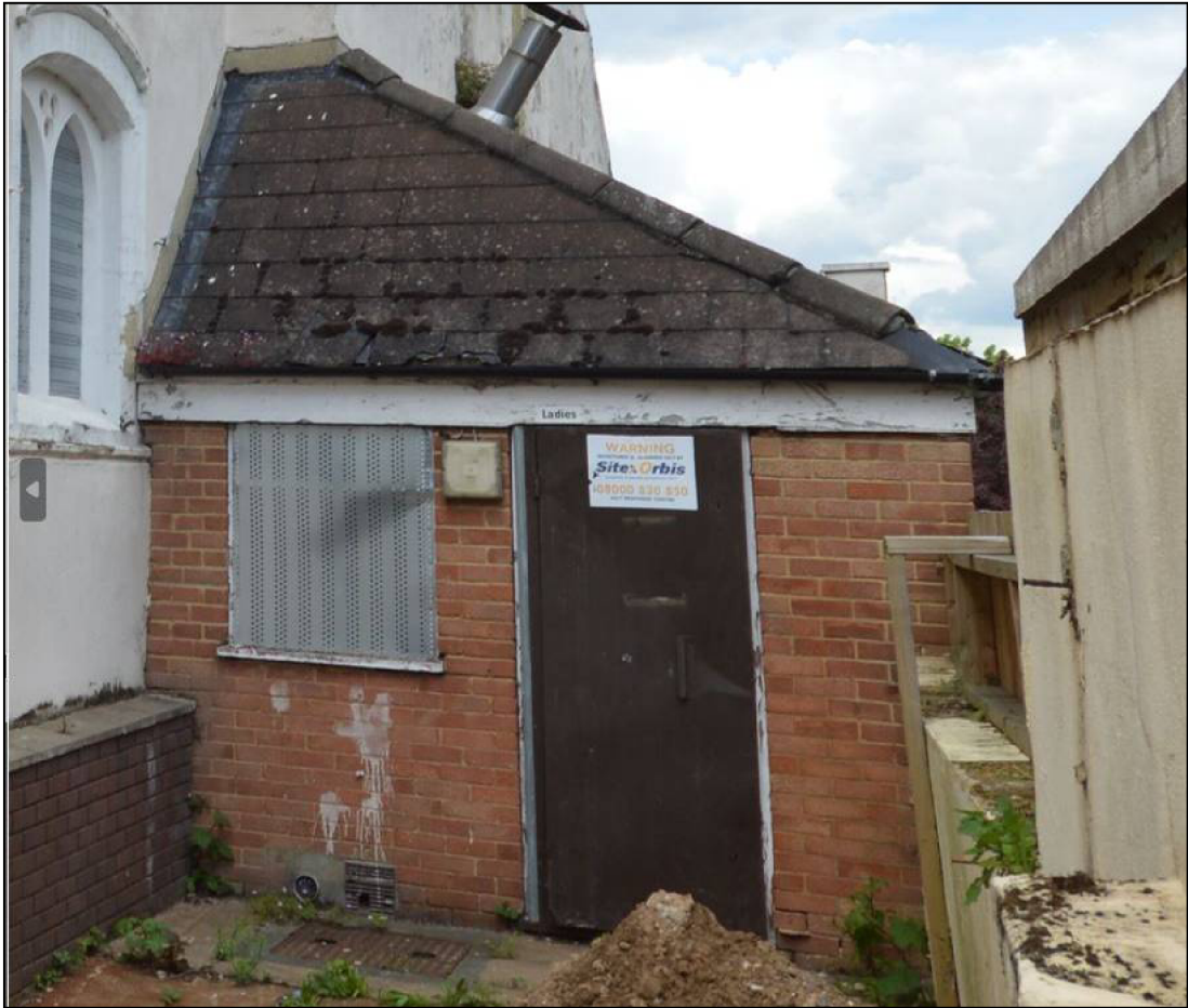
Plate 56: The south elevation of the porch added in 1982
