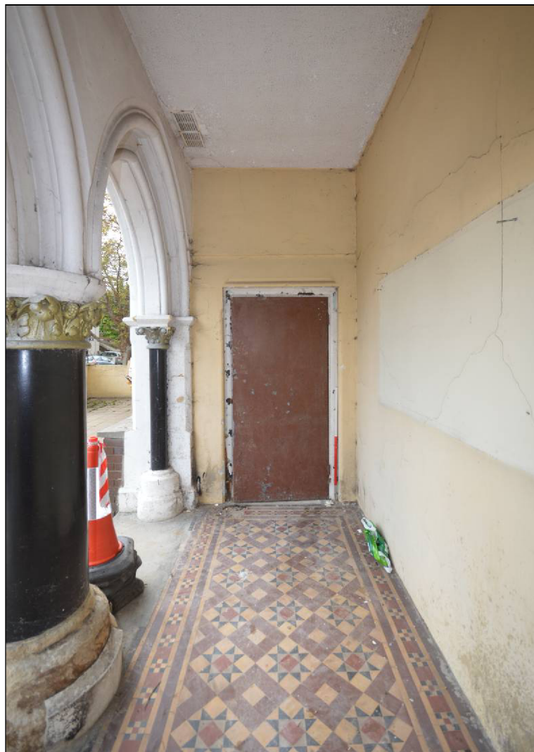
Plate 23: The entrance arcade, tiled floor and western entrance
