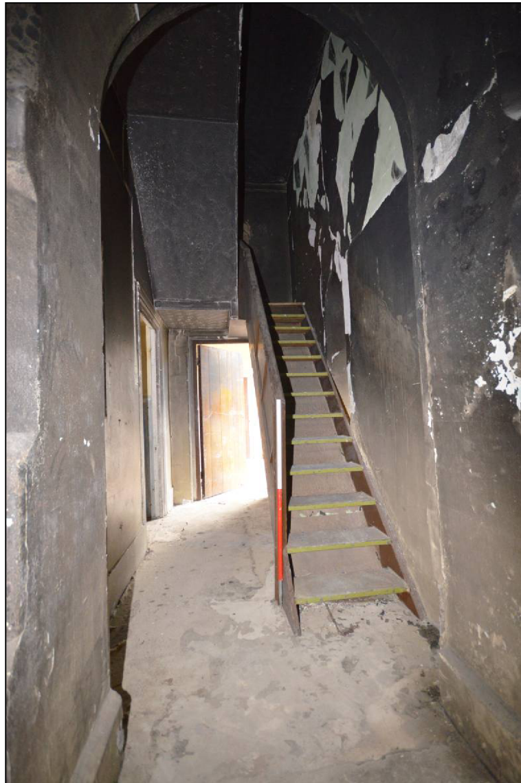
Plate 24: Interior of the west lobby and staircase leading to the south gallery
