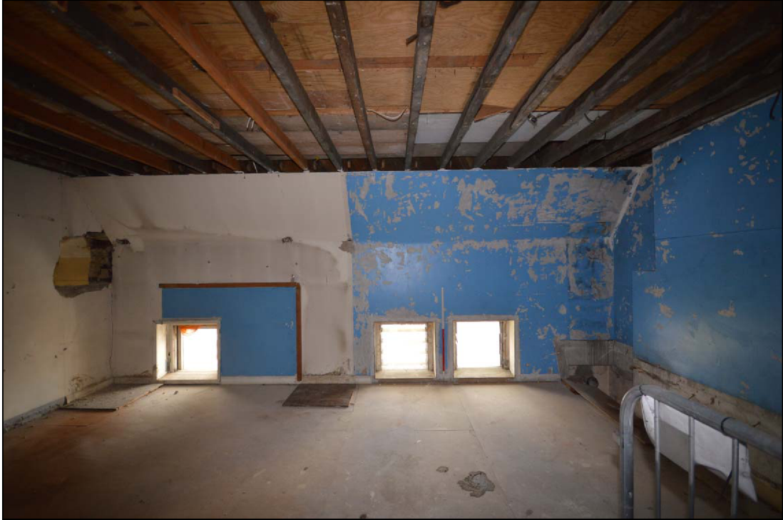
Plate 45: The north wall of the first floor accommodation at the east end of the school house created in recent years
