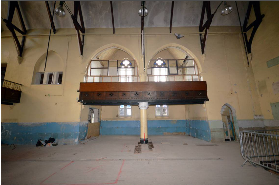
Plate 30: The west aisle arcade and the blocked high-set window to the south of it illustrating the extent of natural light that would have suffused the church at the date of construction
