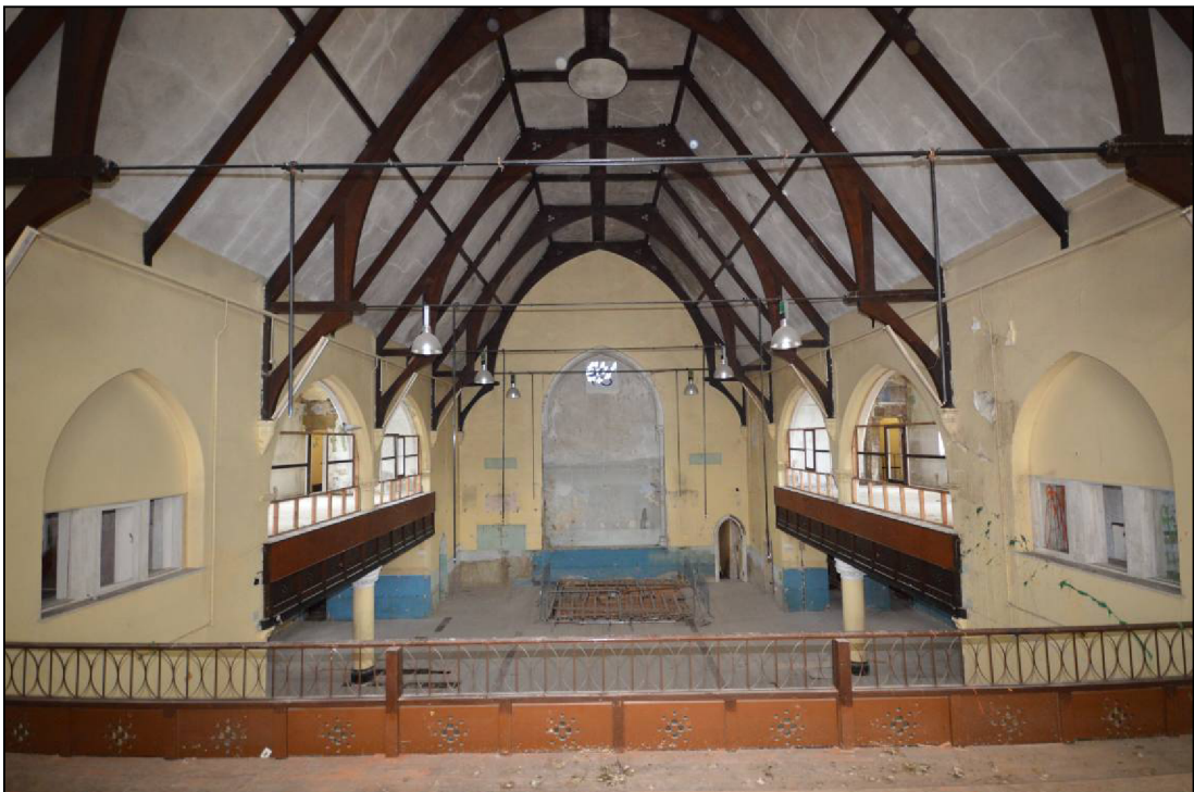
Plate 35: The interior of the church showing the galleries and the roof and ceiling construction
