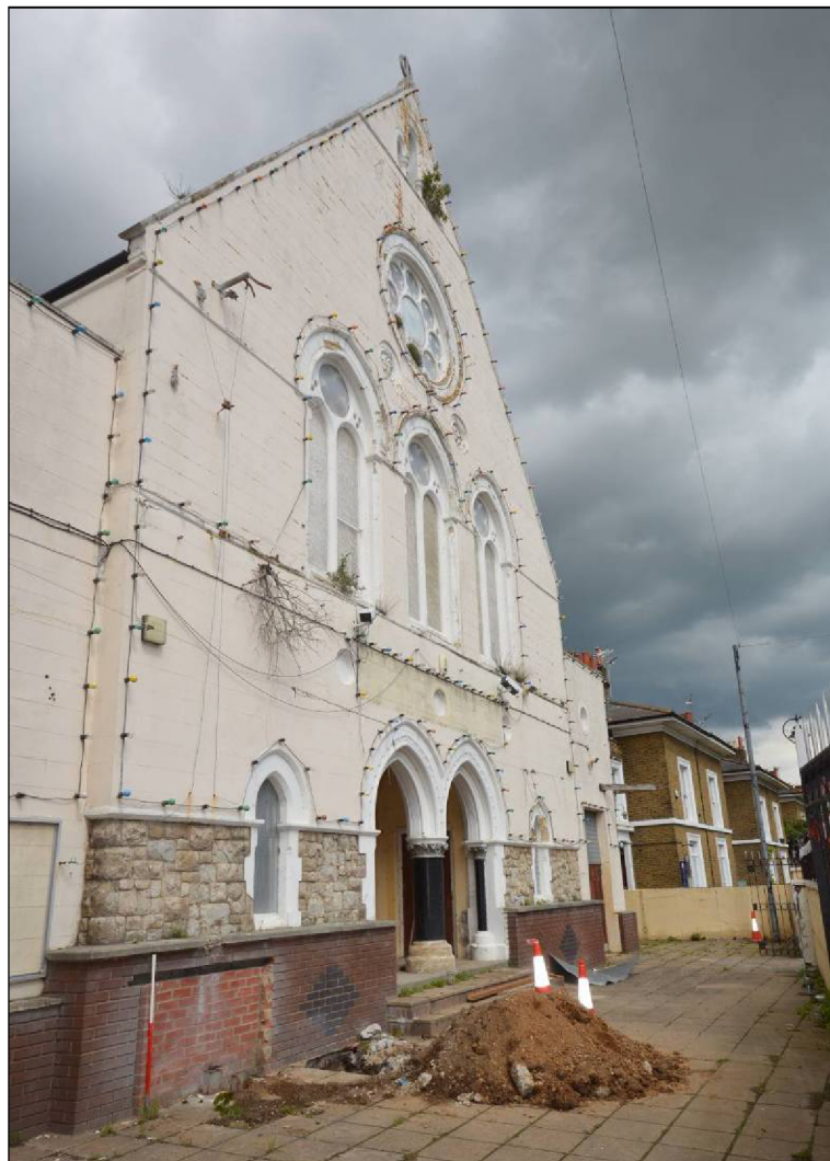
Plate 9: The front (south) elevation of the church looking northeast (scale 1.00 metres)
