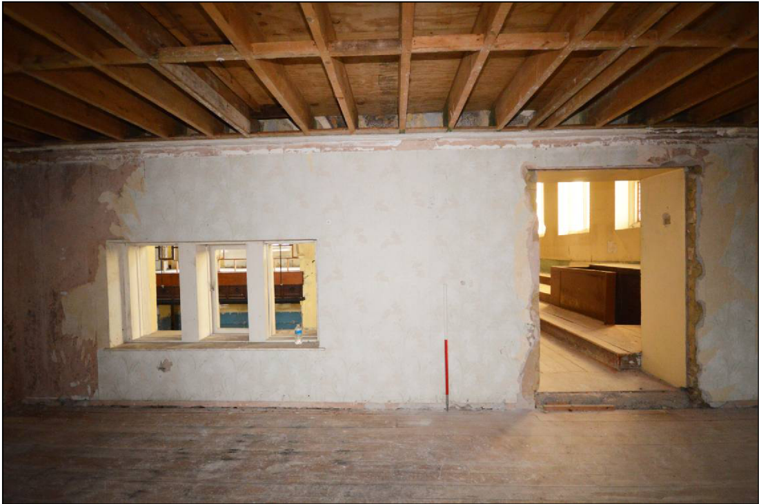
Plate 61: The east wall of the southwest extension; the three-light window is within infill of an original larger high-set pointed-arch-headed window lighting the nave to the north of the south gallery. The doorway was inserted, replacing part of the tripartite window that had occupied that position prior to extension
