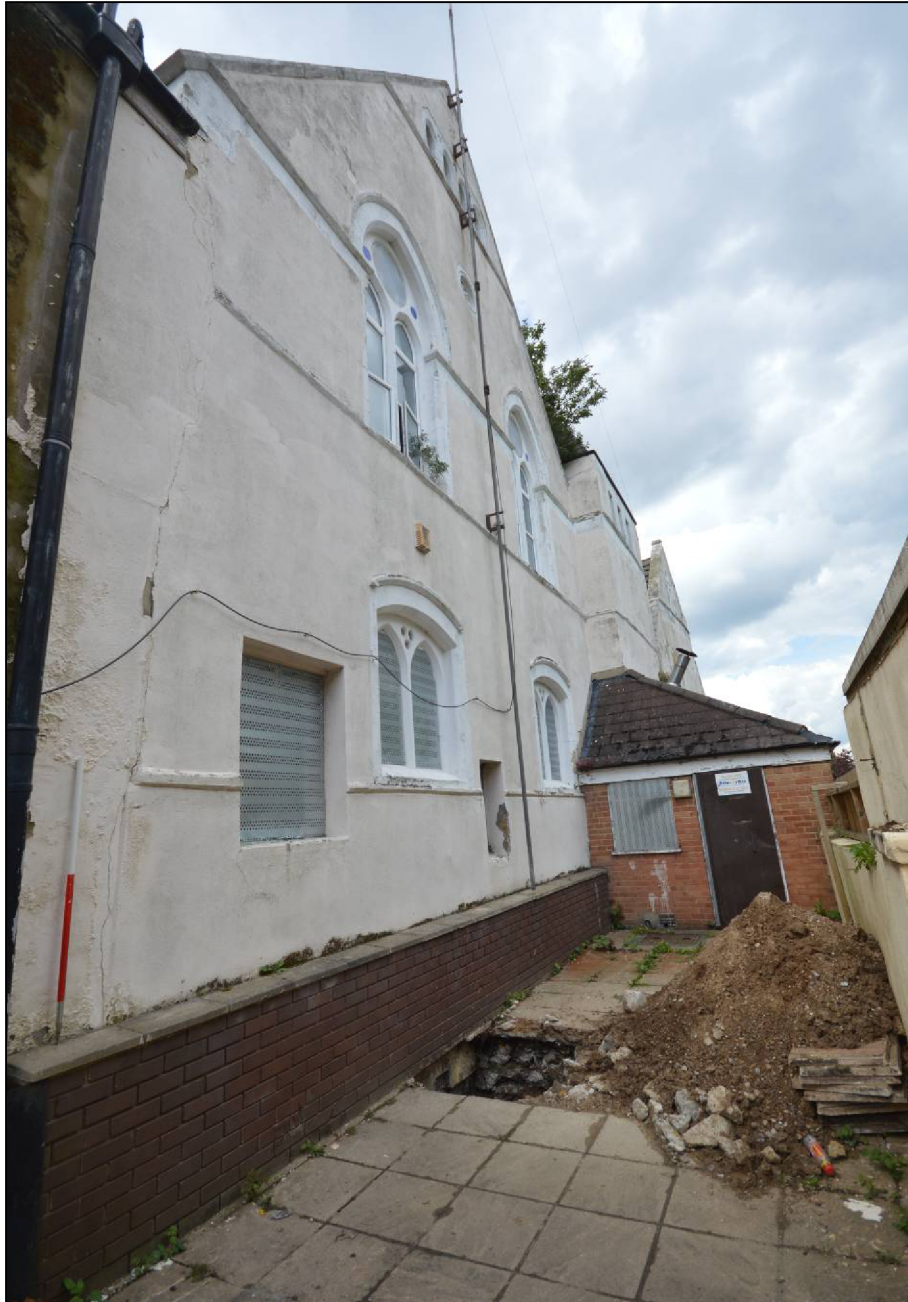
Plate 16: The east elevation and the porch added in 1982
