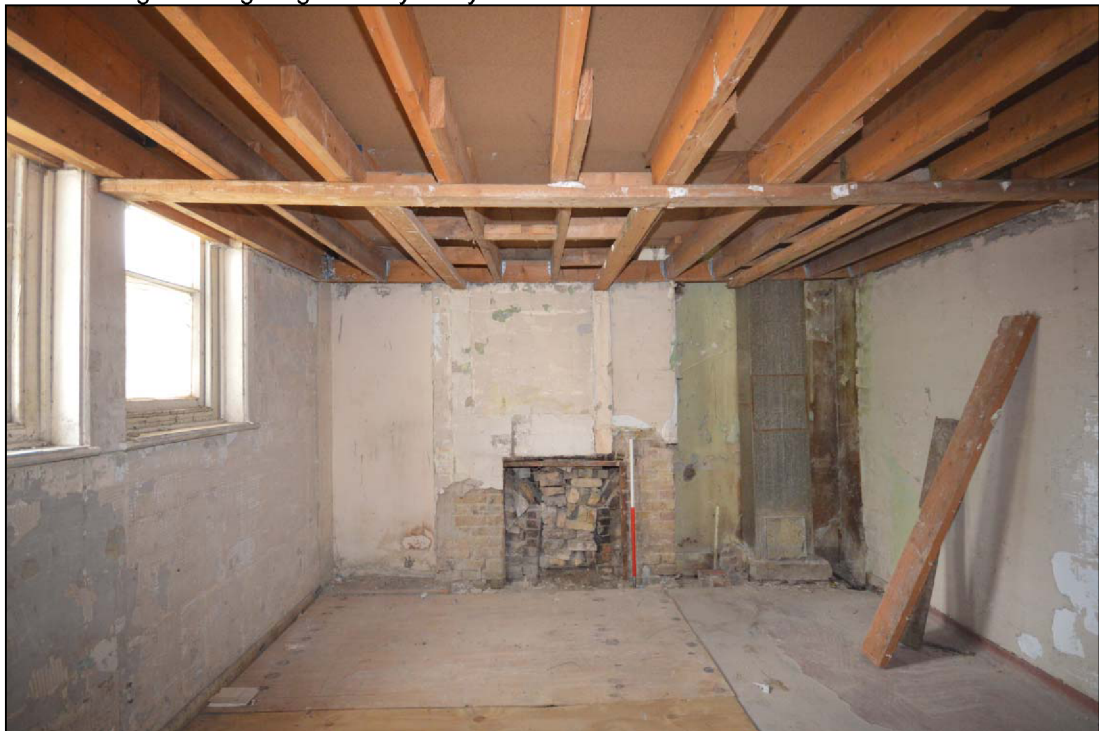
Plate 44: The northeastern room of the school house with its fireplace and windows bisected by the inserted floor structure
