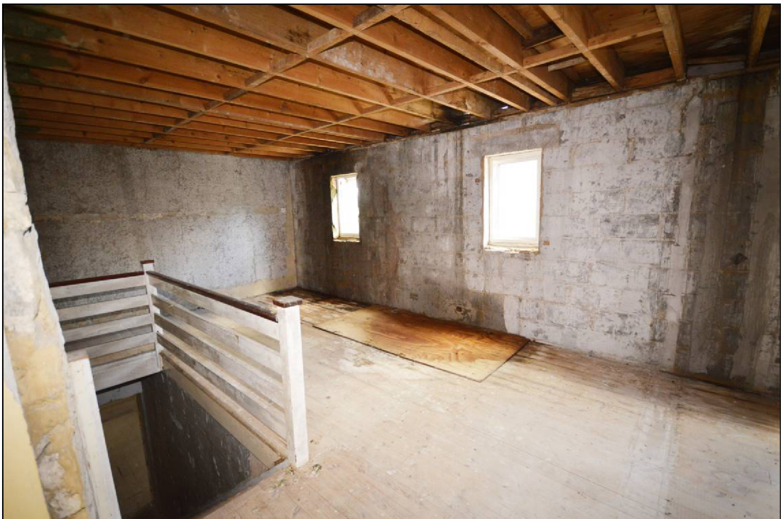
Plate 62: The interior of the southeast extension with its integral staircase in the northwest corner
