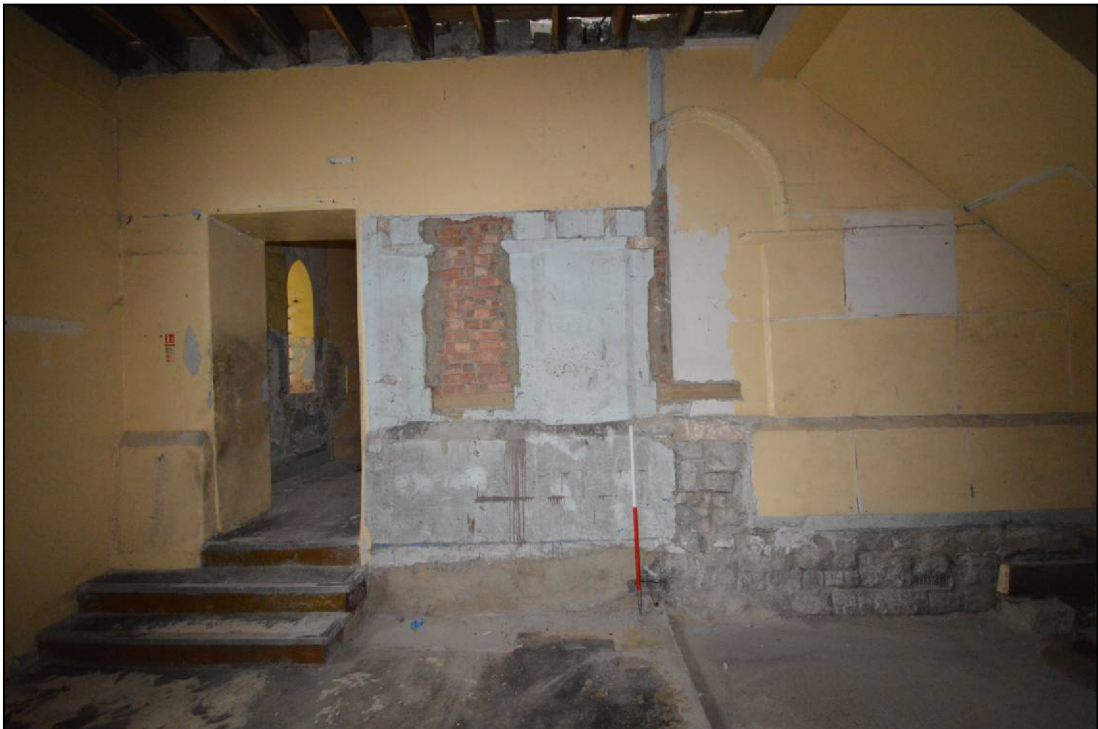
Plate 26: the inserted doorway in the east elevation of the east lobby, viewed from the extension added in 1955
