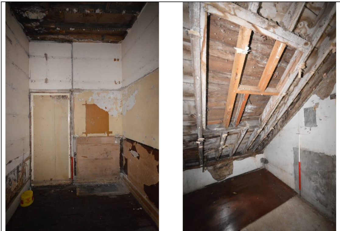
Plate 38: The blocked fireplace in the north wall of the former minister's vestry at the base of the east stair turret and the blocked rooflight in the chamber above
