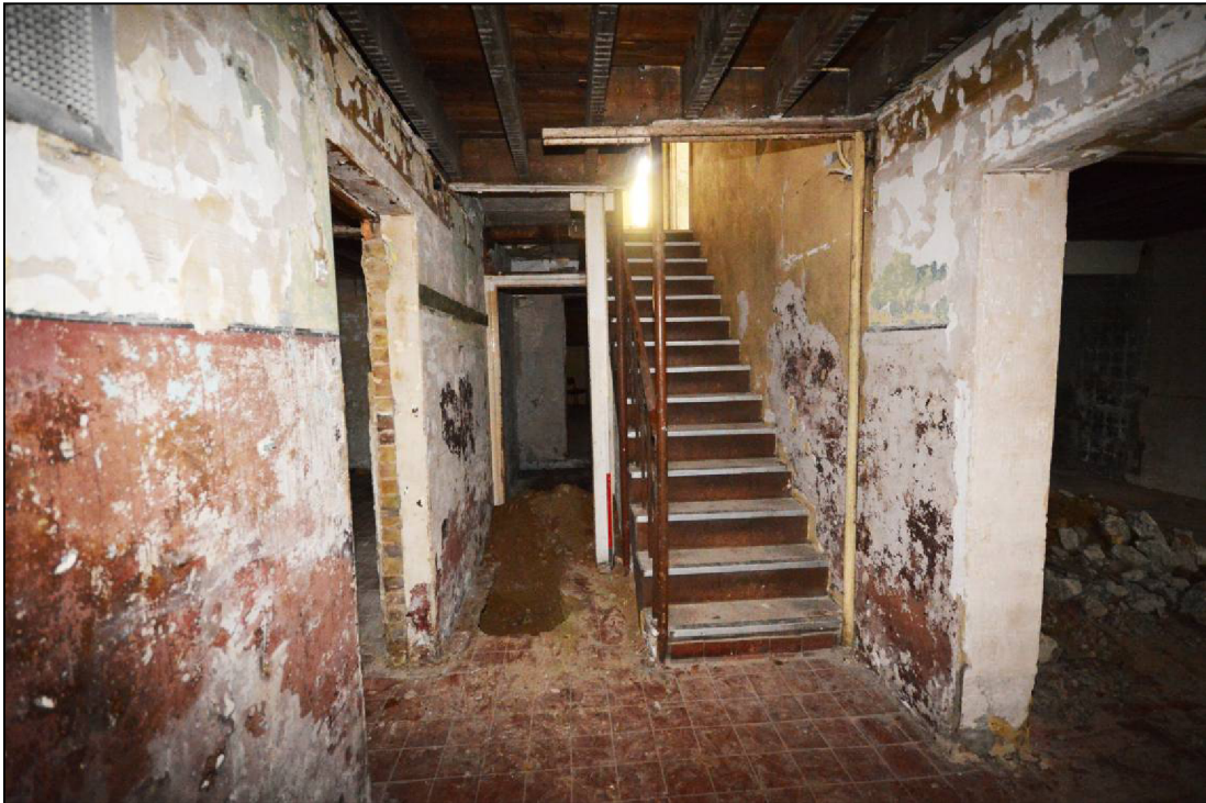
Plate 47: The interior of the stair hall looking south
