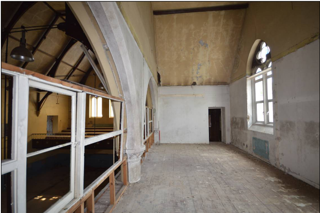
Plate 33: The north end of the west aisle showing the later alterations to the arcade and the doorway inserted to create access to the 1975 extension
