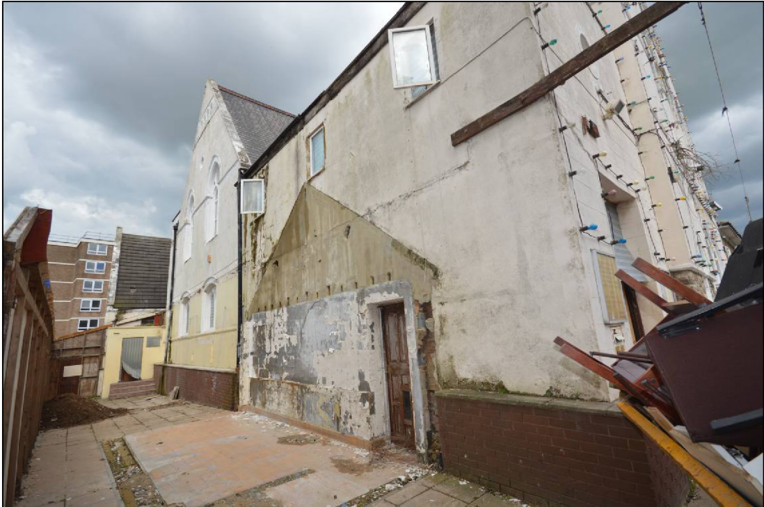
Plate 21: The southwest extension and the scars left by the addition made in 1982 to accommodate new WC facilities
