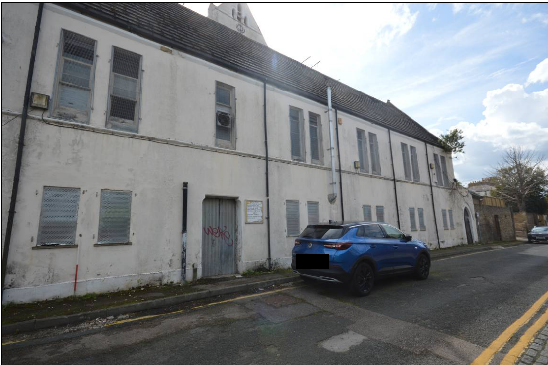
Plate 12: An oblique view of the north elevation as existing in 2023
