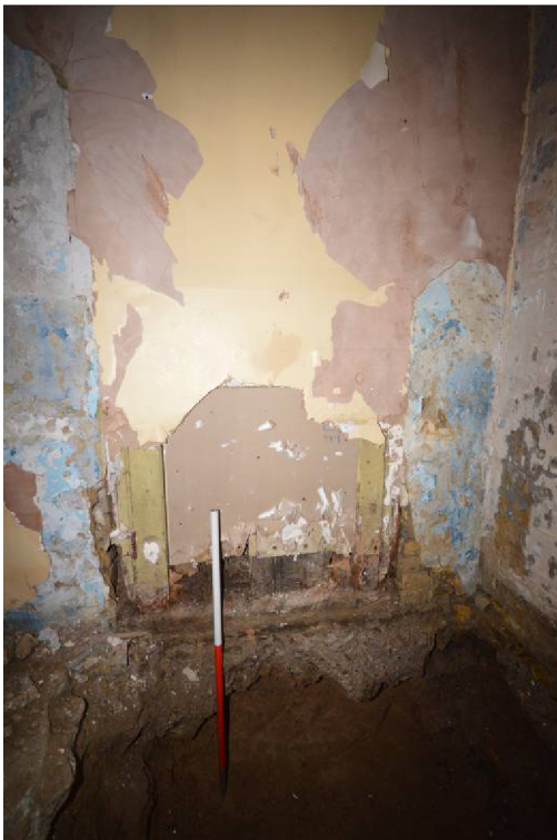
Plate 51: Detail of the blocked doorway showing the timber-frame in situ
