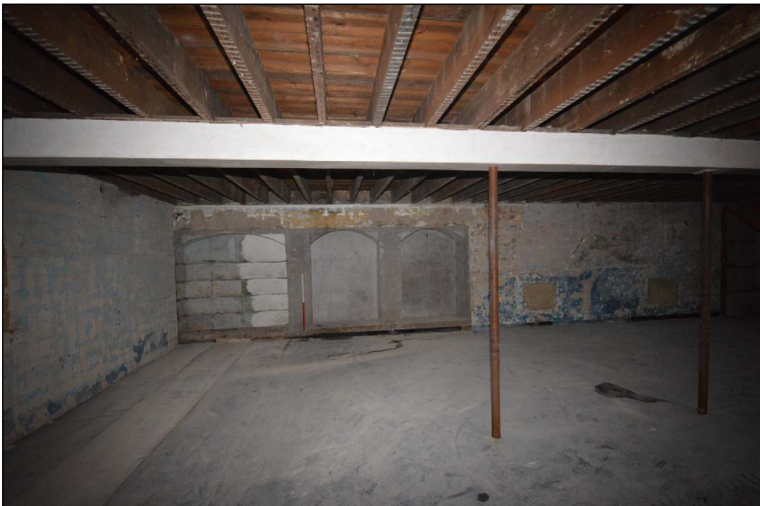
Plate 49: The lower ground floor west classroom looking south showing the series of niches integral to the wall in that location
