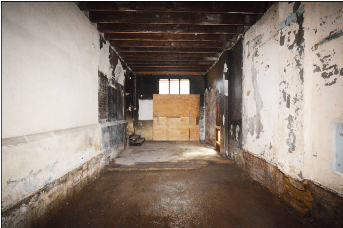
Plate 58: The interior of the southwest extension on the ground floor, looking south
