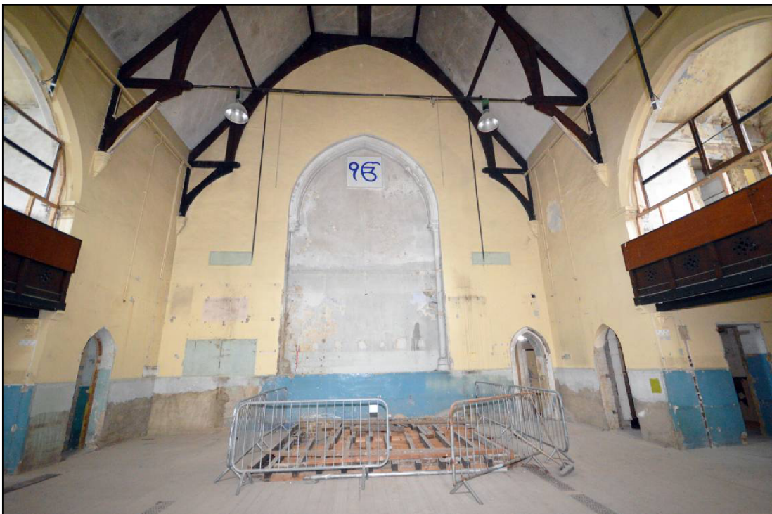
Plate 28: The north end of the nave with the remains of the platform and the recess that had framed the organ
