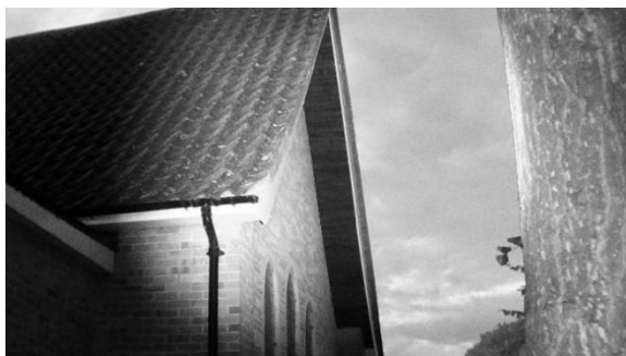
Screenshot from building B9 camera (25/08/23).
