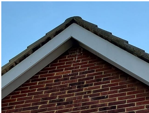
The northern gable end of building B7.
