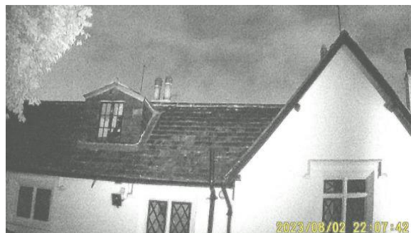
Screenshot from building B10 camera (02/08/23).
