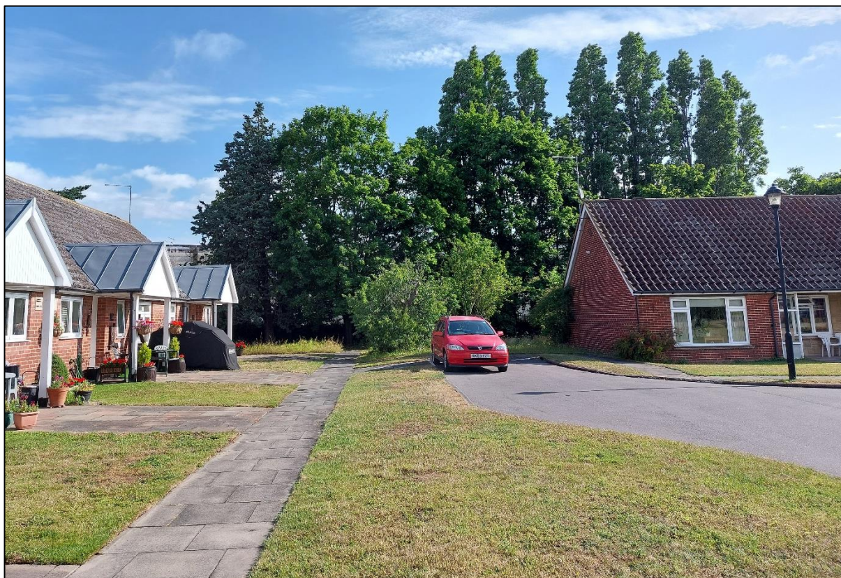
The northern boundary (July 2023), showing the poplars, chestnuts and three fruit trees due to be removed (in the foreground).
