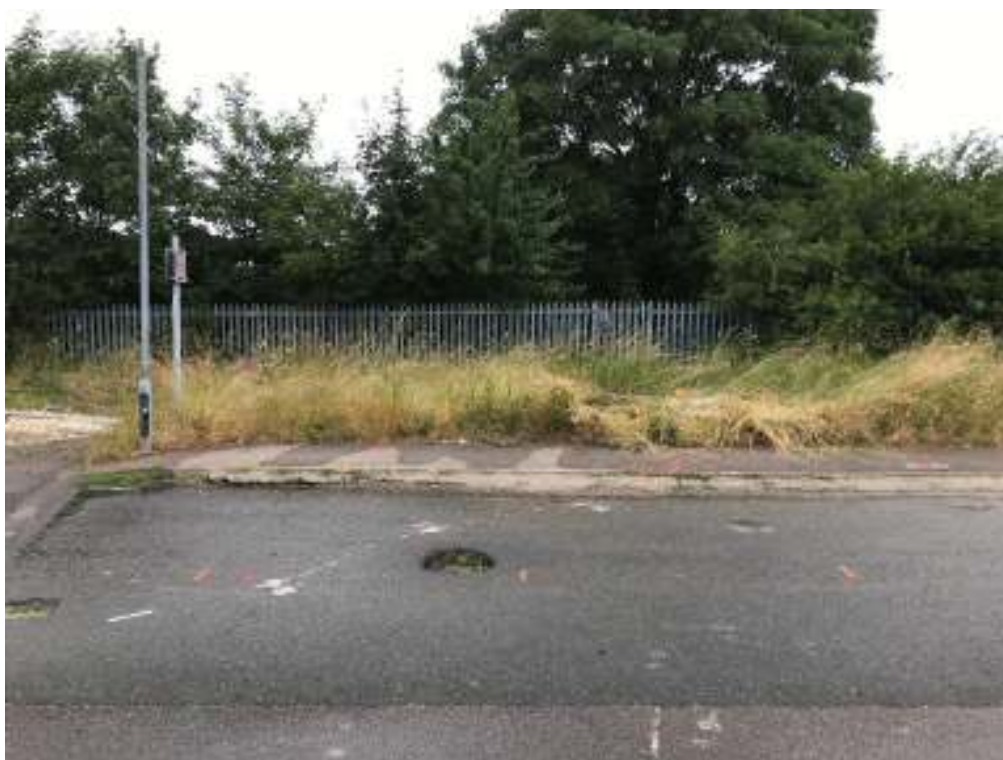
2 nd July 2024 – Soft landscaped area on northeast of site, looking north
