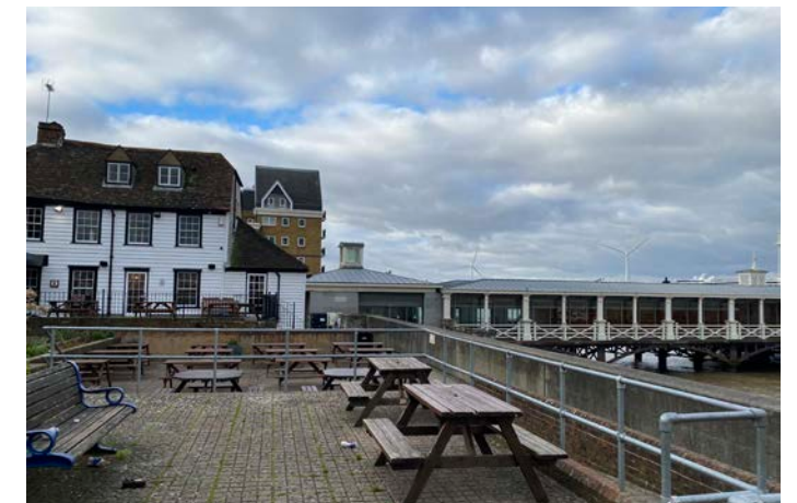
Figure 4.9 Town Pier viewed from the west of the mooring point Site Visit 2024
