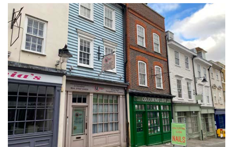
Figure 3.14 Historic weather boarded houses on High Street Site Visit 2024
