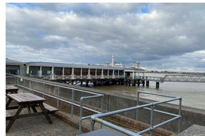
Figure 4.11 The pier extension viewed from west of the mooring point Site Visit 2024
