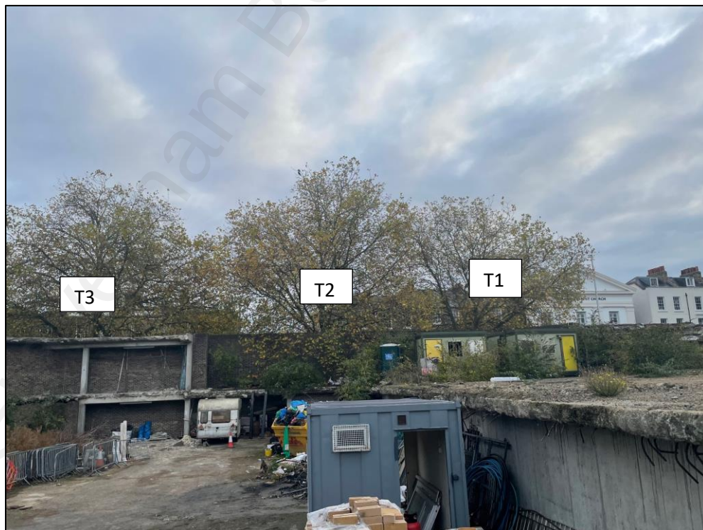
Photo 2: Looking at trees T1, T2, and T3 from inside the site. The existing structure is currently being demolished and the boundary brick element can be seen. Pruning is proposed to reduce the lateral branches overhanging the site.
