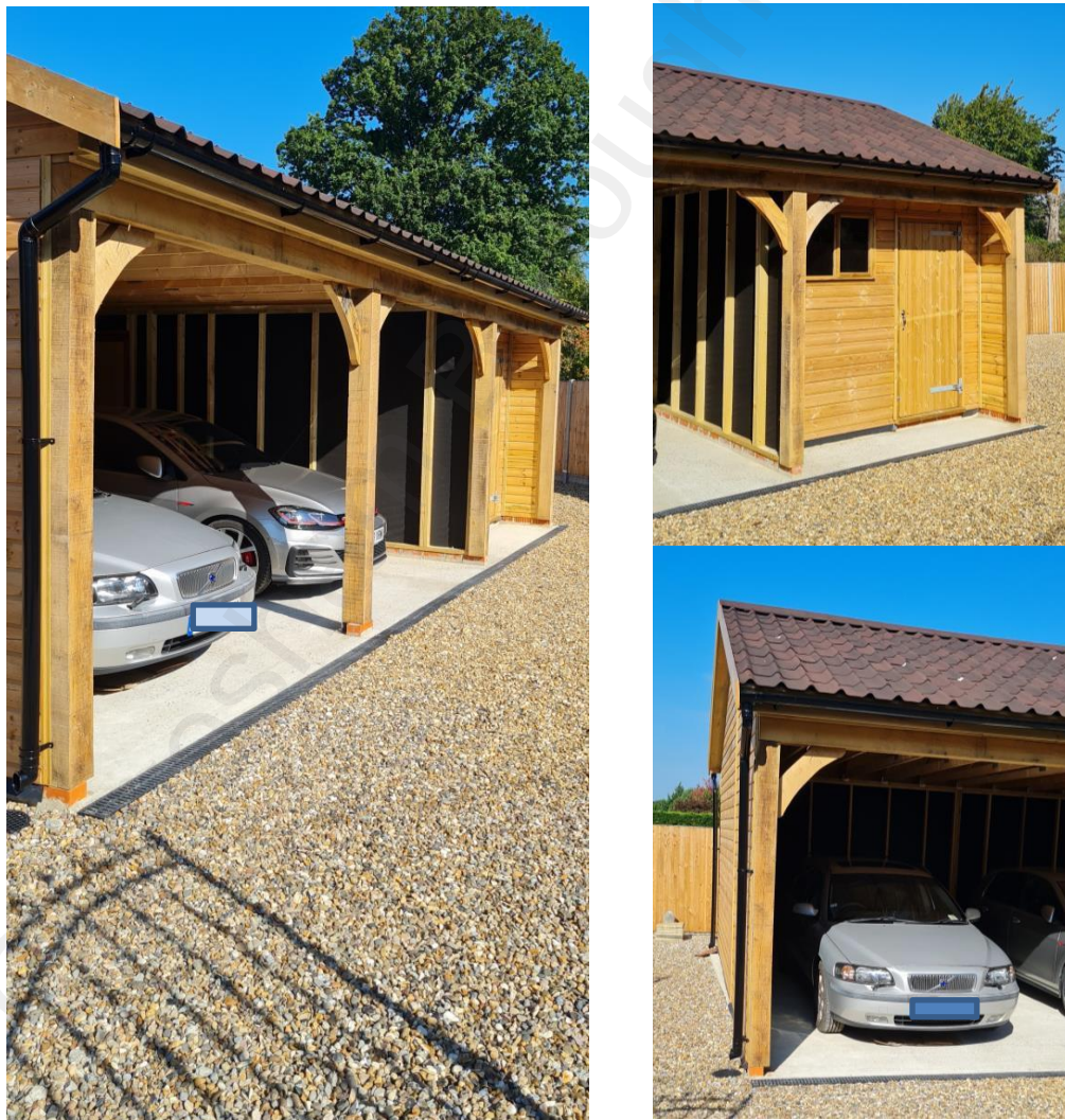
Photograph 1 -3: Photograph showing the garage building
