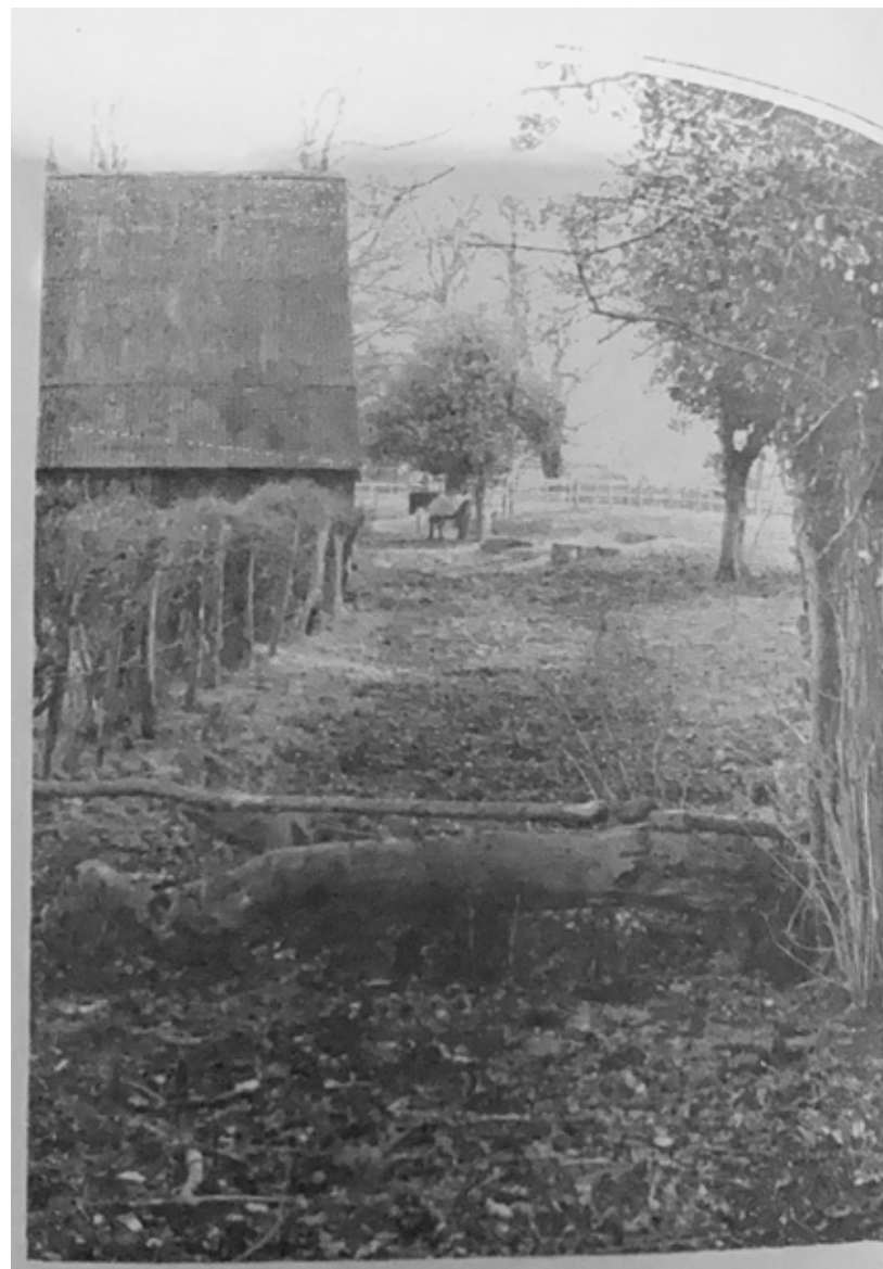
Historical photo - Norwood Lane adjacent to the south gable wall
