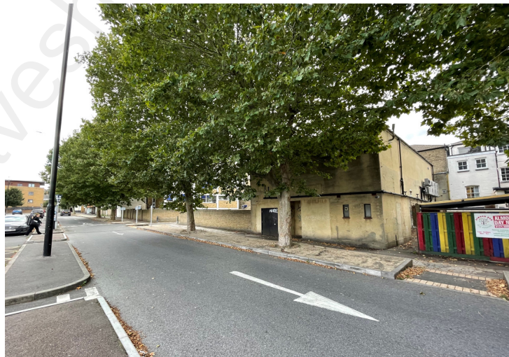
Rear of 44 Windmill Street
