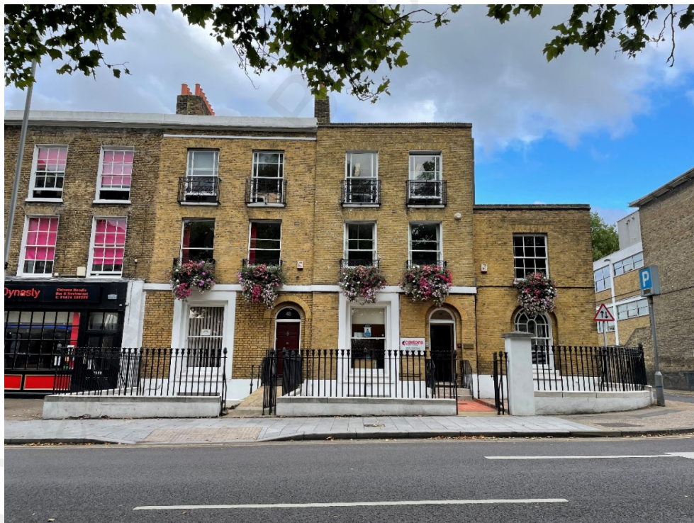
Number 49, 50 within Listed Terrace 38-50 Windmill Street
