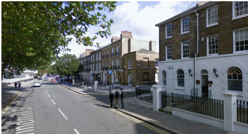
49 – 50 Windmill Street junction with North Street
