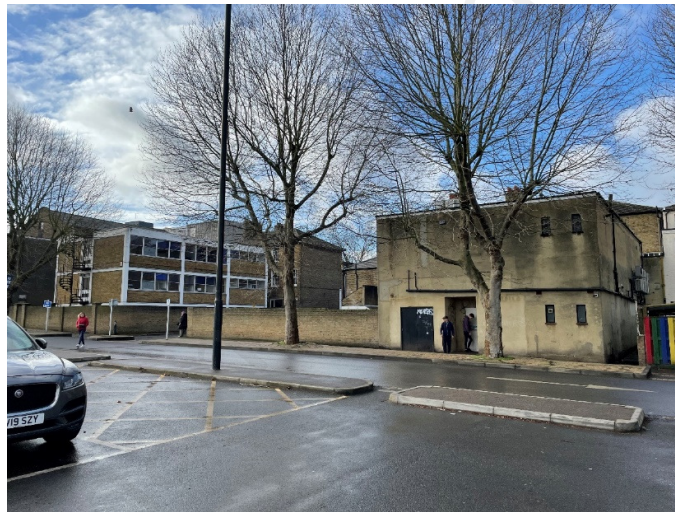
Fig 6 – Rear of site
