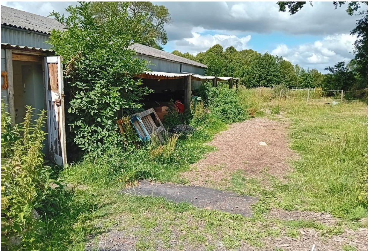
The existing building and surrounding grassland.
