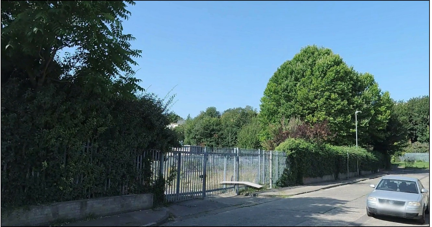
Google earth image from Crete Hall Road, facing into the site.
