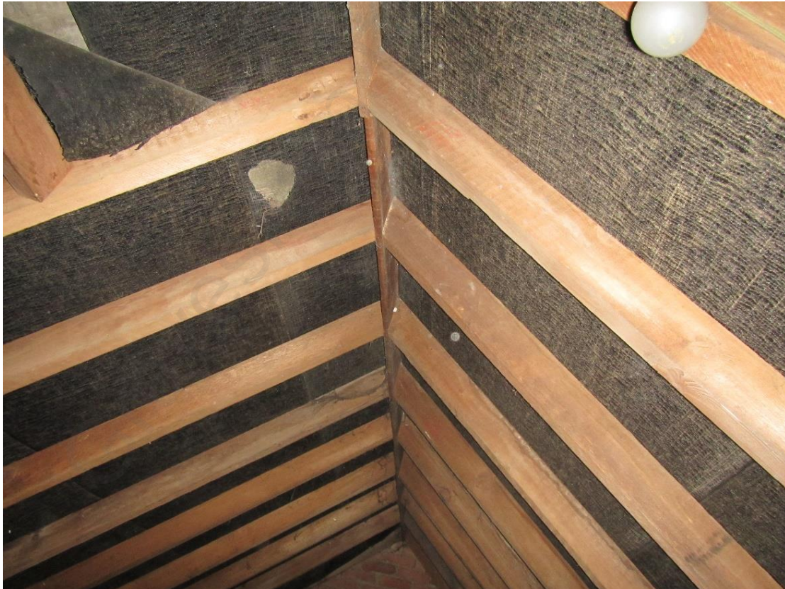
Photograph 8 – The underside of the roof is lined with bitumen roofing felt.
