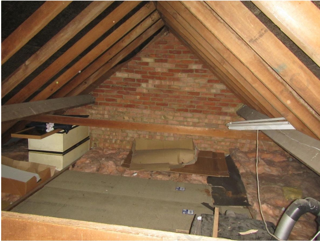
Photograph 7 – View of the loft void.
