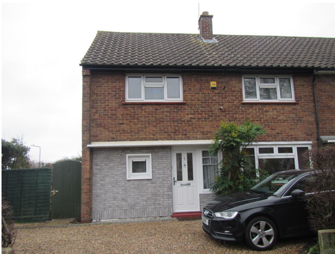
Photograph 7 – Looking east towards Building 1, an end-terrace residential dwelling that will be retained as part of the development proposals.
