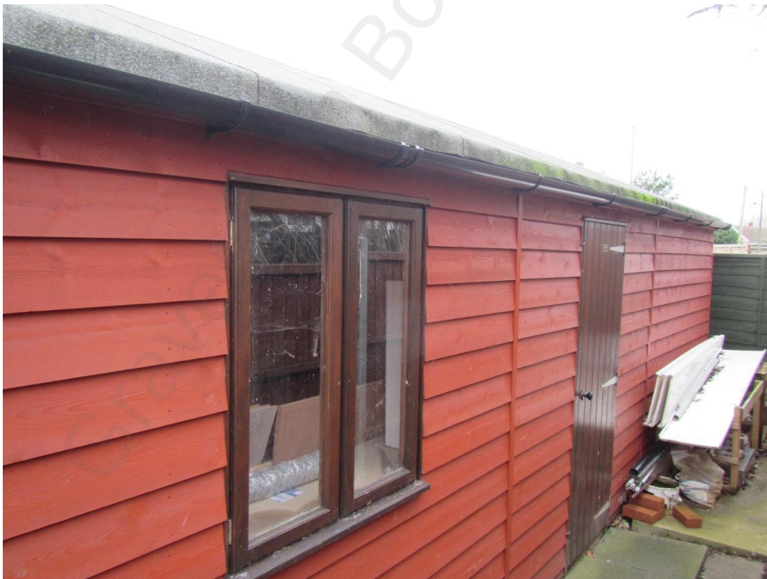
Photograph 10 – Looking towards Building 2, a single-storey shed / out building that will be retained as part of the proposals.
