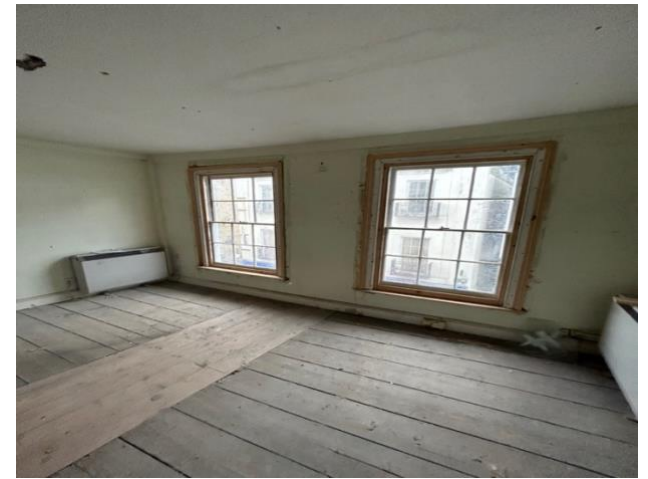
Fig 12: Sash windows on the first floor
