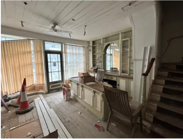
Fig 7: Showing ground floor with staircase floor
