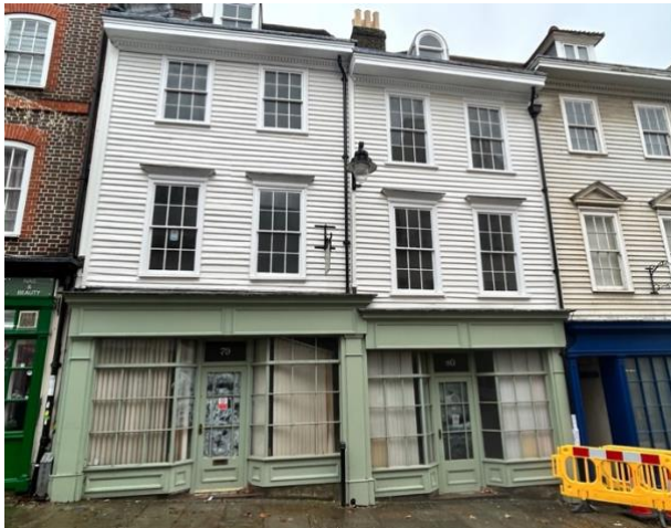
Fig 19: High Street frontage
