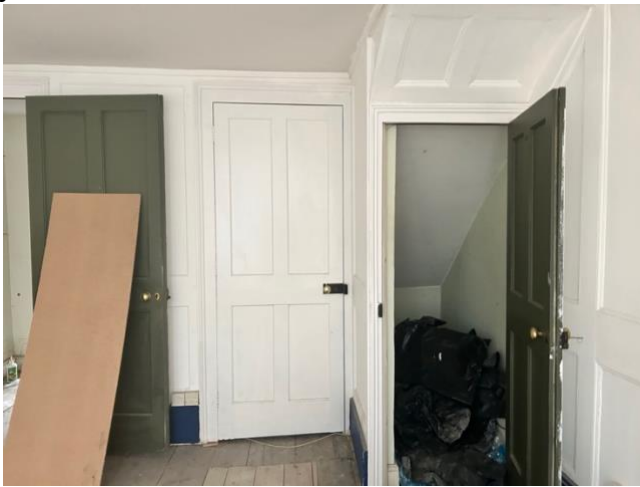
Fig 9: The existing doors on the first floor
