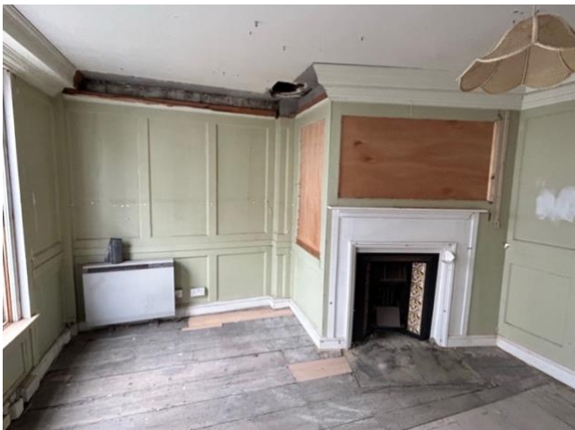
Fig 11: First floor with panelling and fireplace
