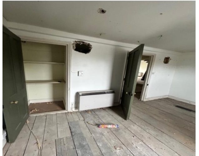
Fig 14: First floor showing modern fittings
