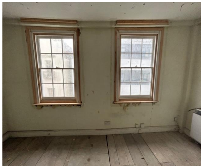
Fig 18: Timber sash windows
