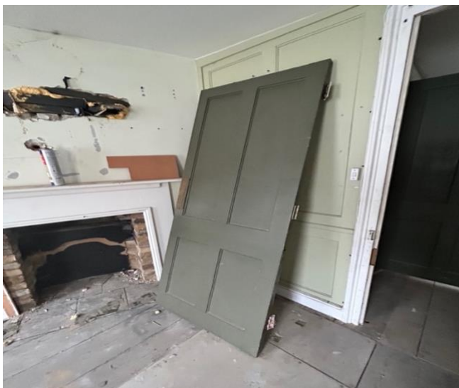
Fig 17: Showing the condition of the interior
