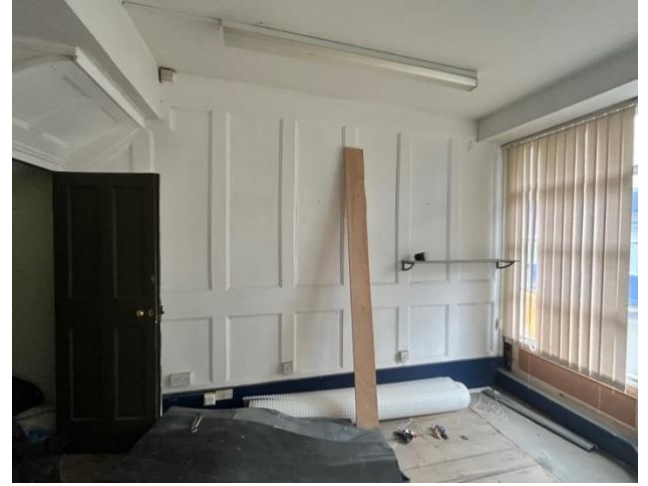
Fig 8: Timber panelling on the ground floor
