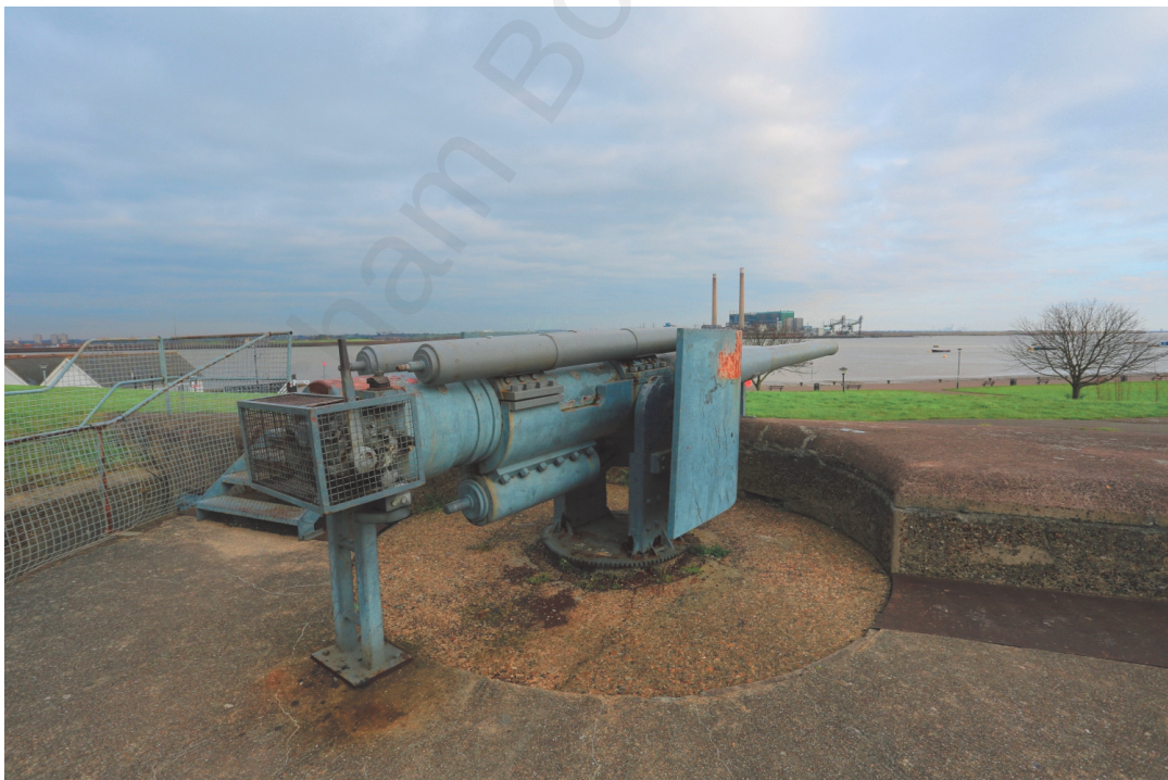
Concrete floor of east gun emplacement
