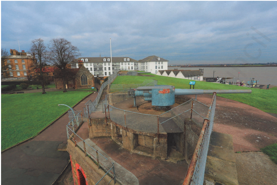
East gun and stores, looking north-west
