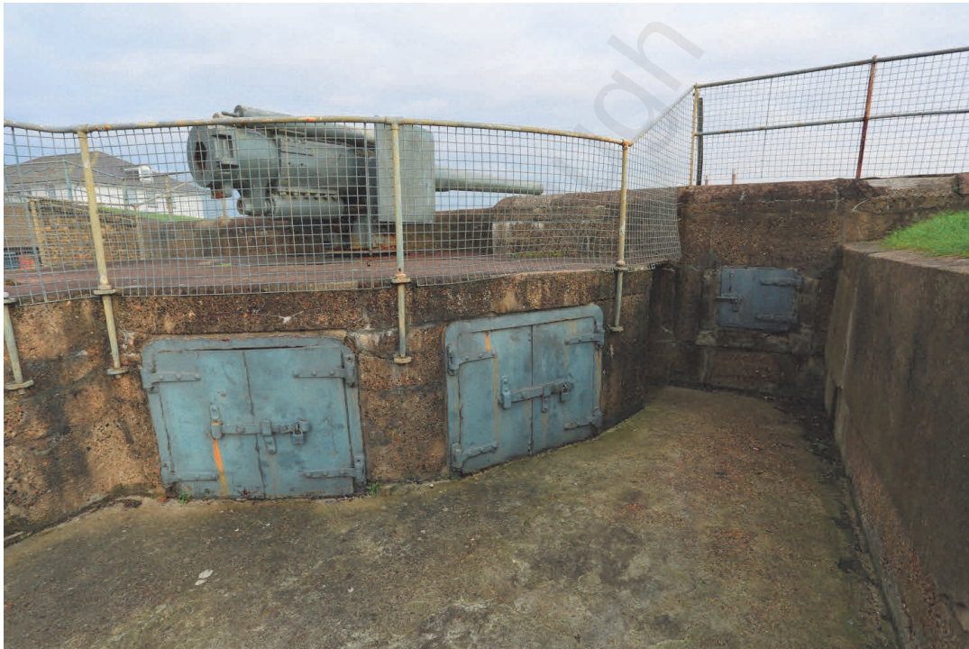
Doors on gun stores of east emplacement
