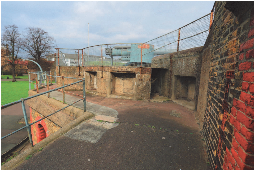
East gun stores, looking west
