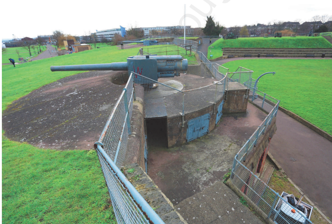
Concrete emplacement of west gun, looking east
