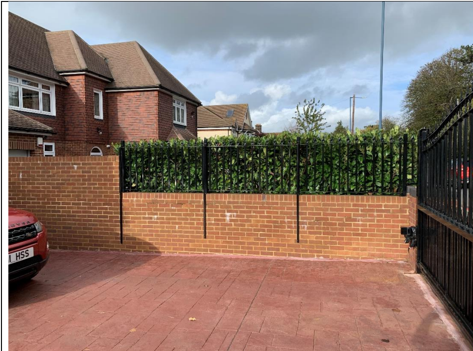
Railings to 369 Singlewell Road
