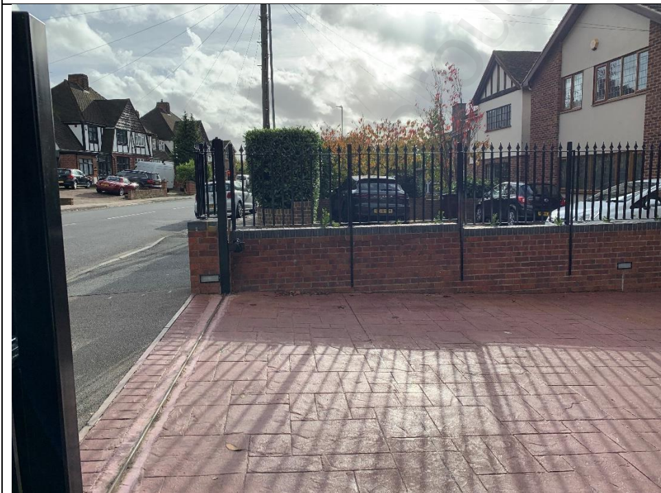
Railings to 373 Singlewell Road
