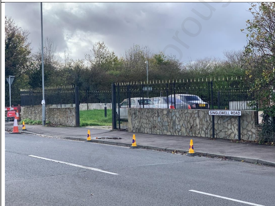
Existing Railings at 377 Singlewell Road
