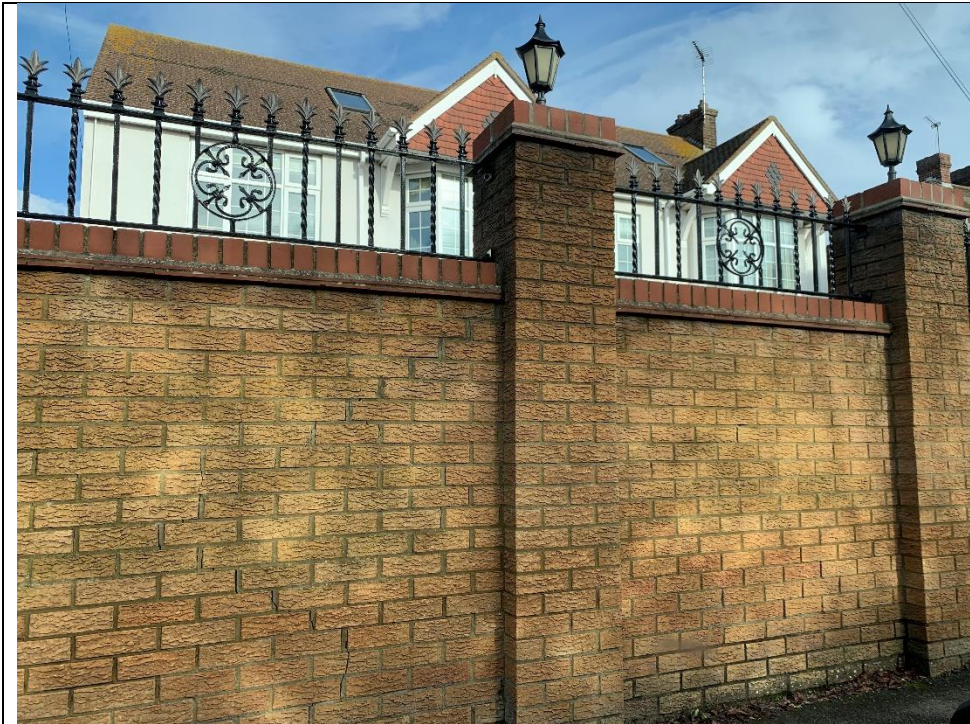
Existing railings, property between Roman Way and Nil Numero
