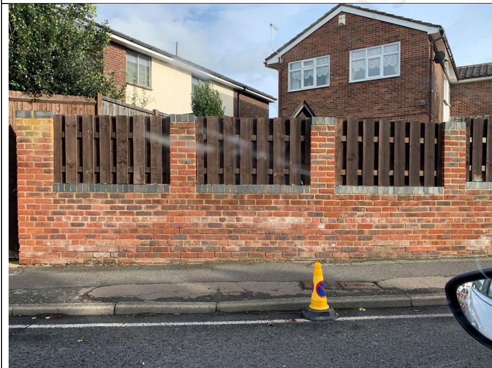
Existing enclosure at 378 Singlewell Road
