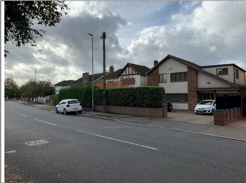
Adjacent Property 373 Singlewell Road
