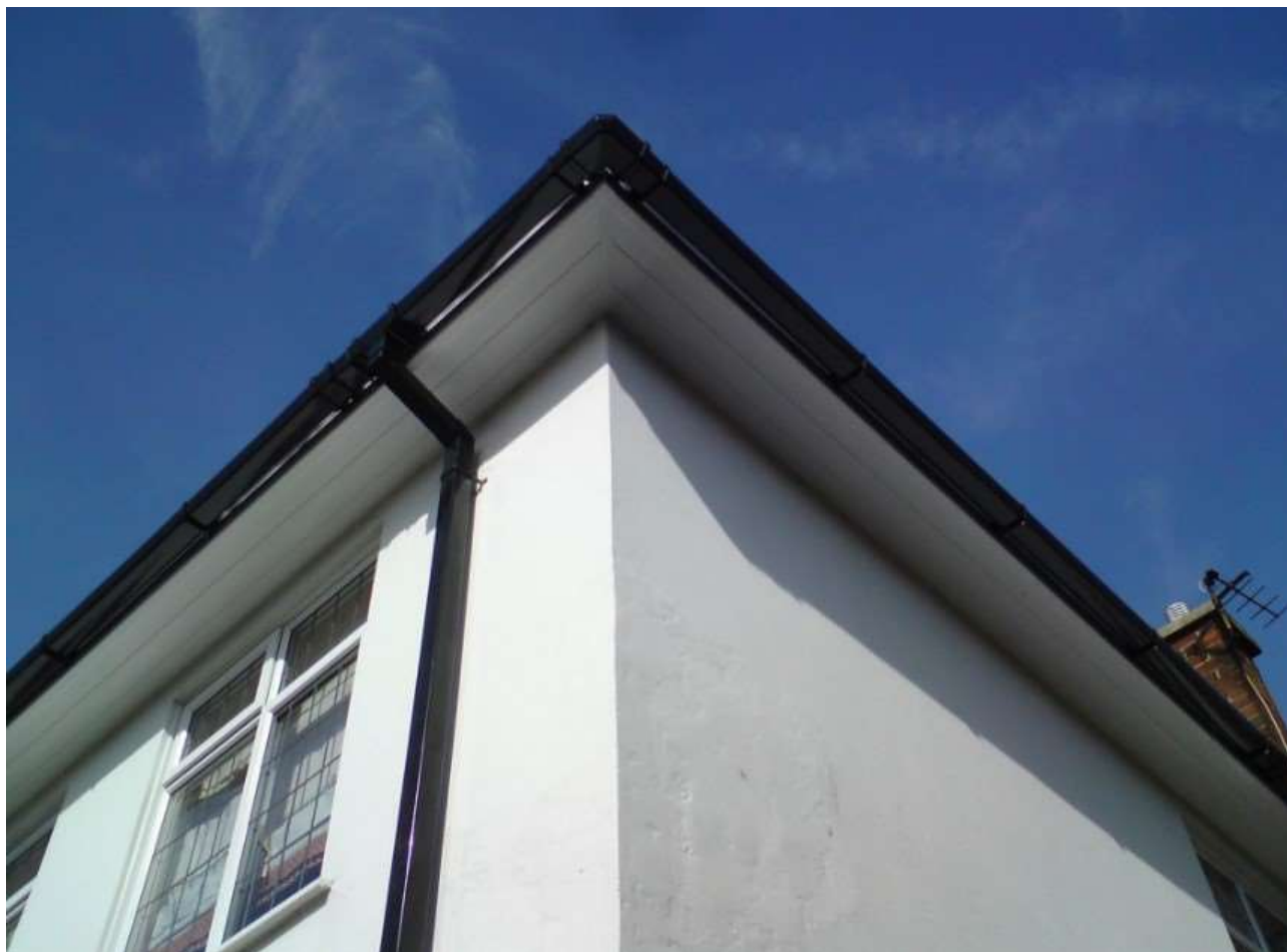
Black upvc guttering and downpipe with white upvc fascia and soffite
