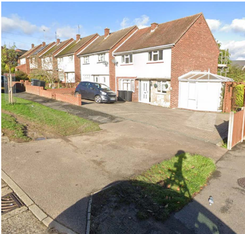
Photo of the existing dropped kerb at no. 60 Livingstone Road
