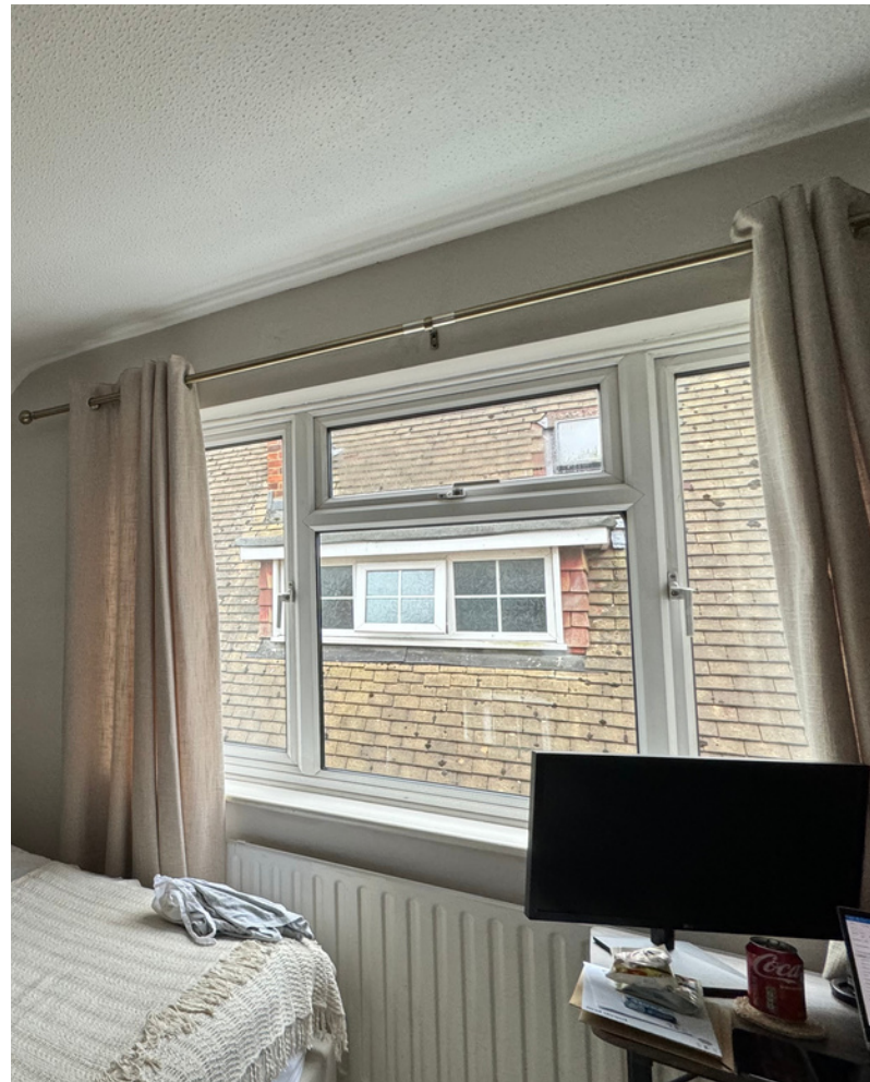
Photo showing existing overlooking window that is being removed in the proposed development
